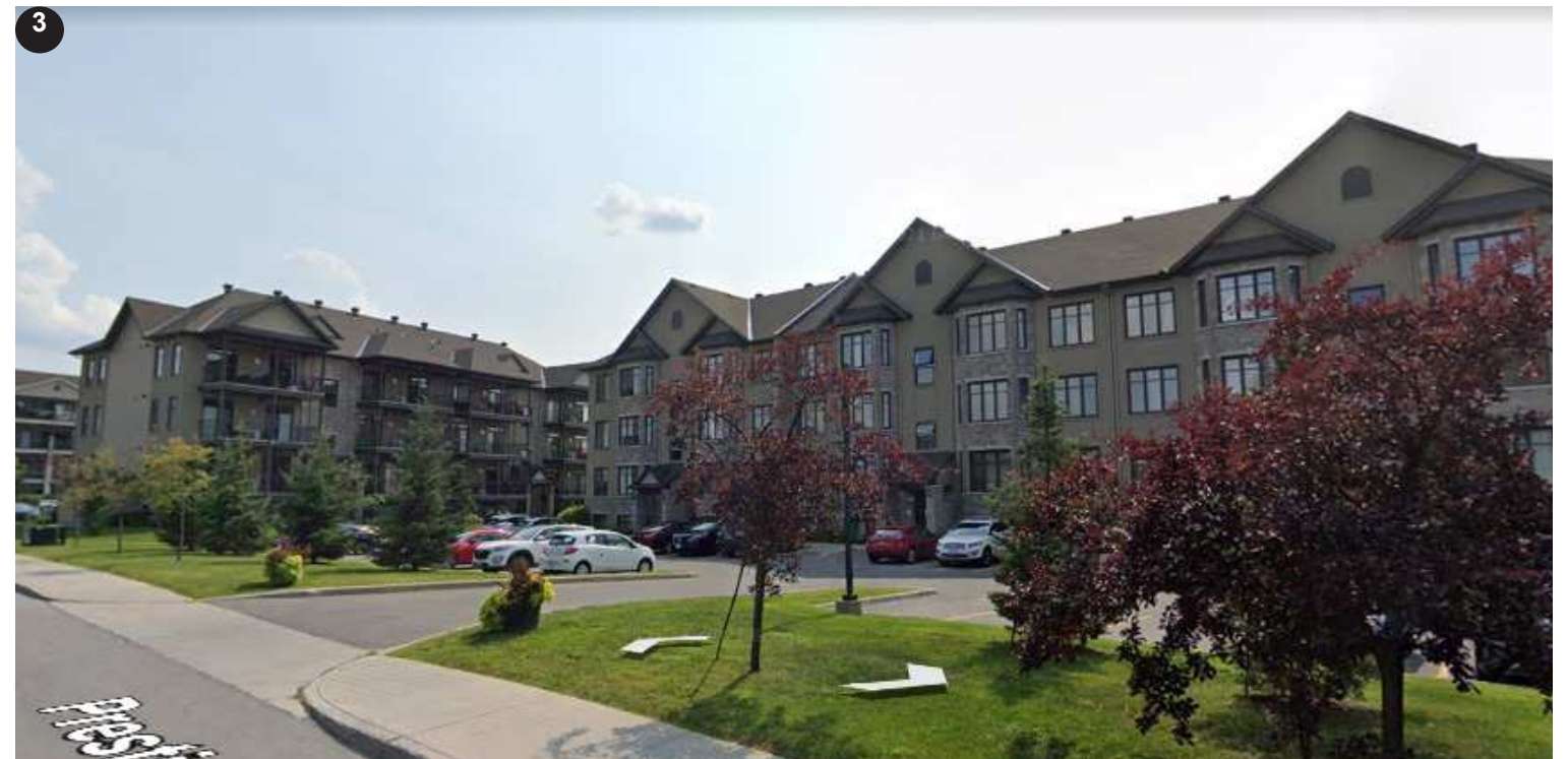
NEIGHBOURING RESIDENTIAL DEVELOPMENT
