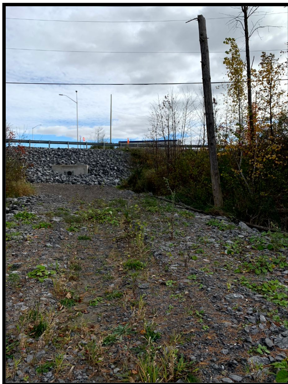
Figure 4: Overview of site with road access (MH1329-D009)
