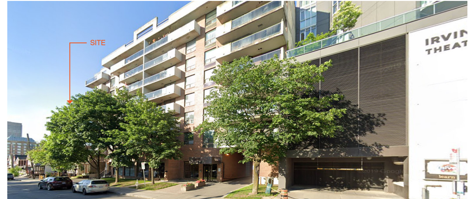
2 - VIEW FROM HOLLAND LOOKING NORTH
