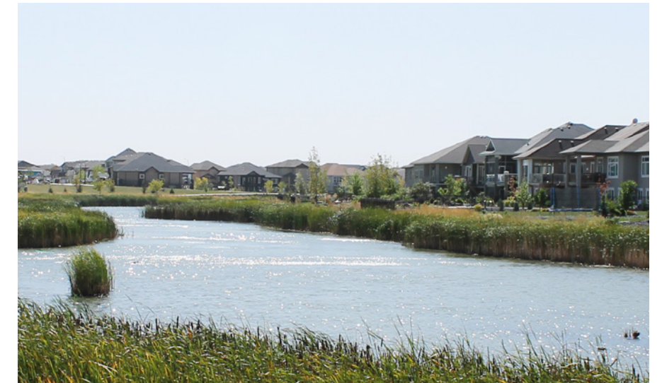
Stormwater Management Pond
