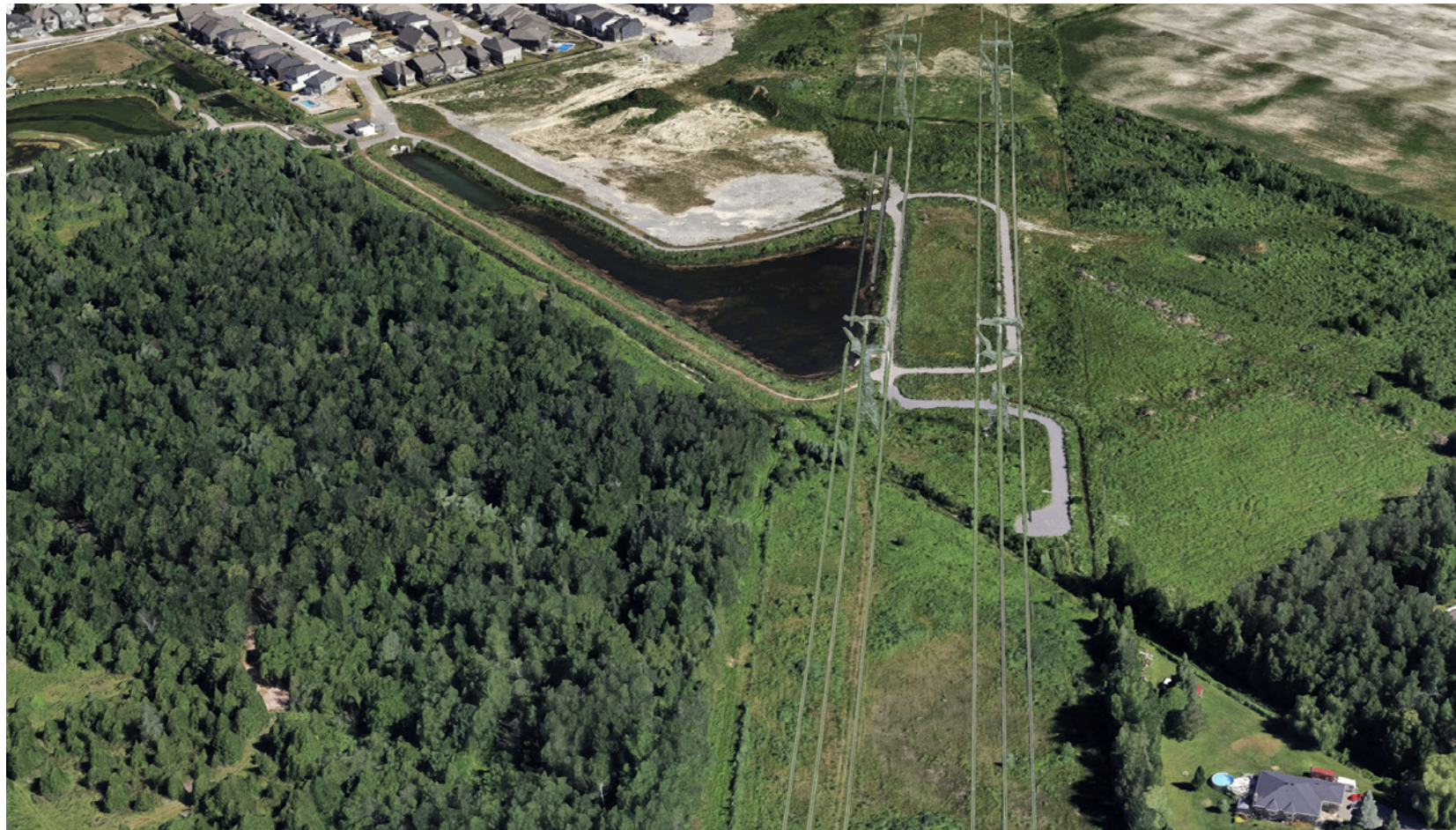
View of Existing Hydro Corridor and Stormwater Management Facility
