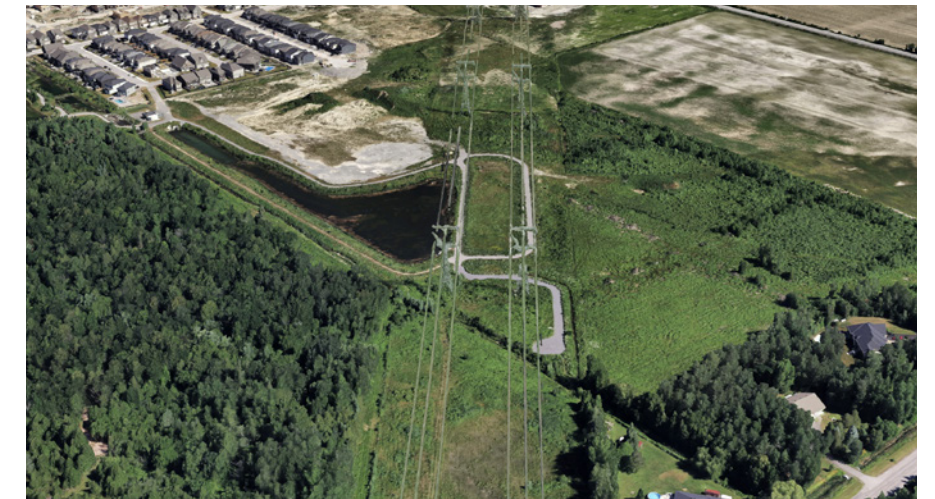
View of the Existing Hydro Corridor
