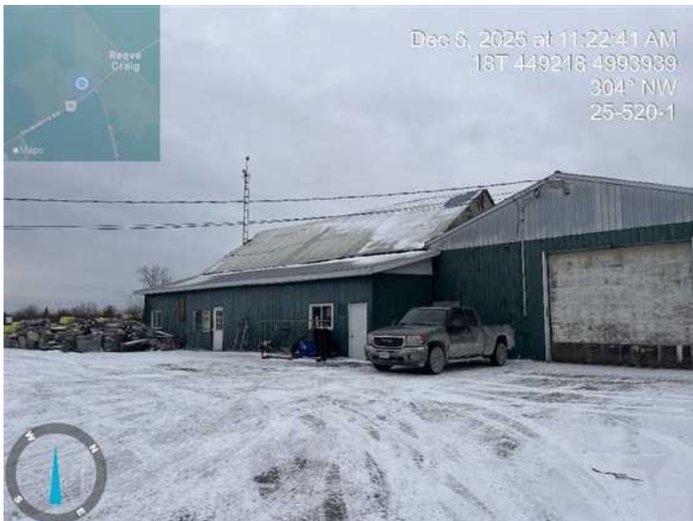
Photograph 16 – View of the commercial service garage.
