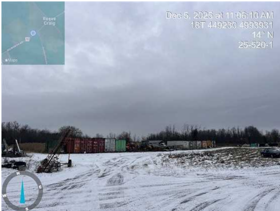
Photograph 5 – View of the metal shipping containers, facing north.
