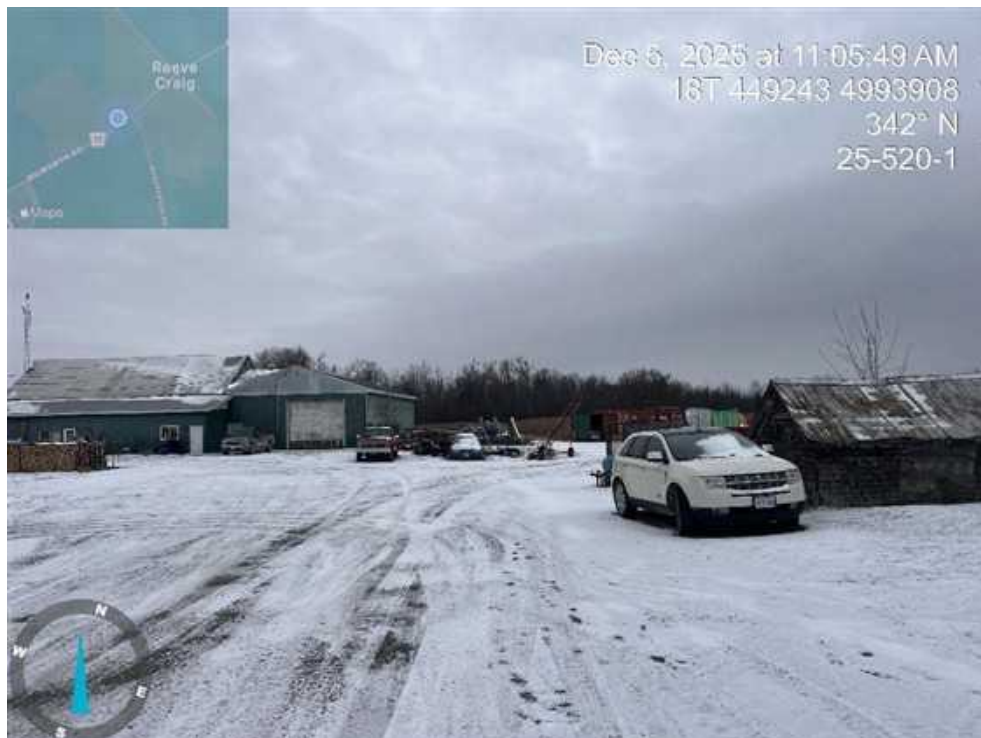
Photograph 4 – View of the commercial service garage.
