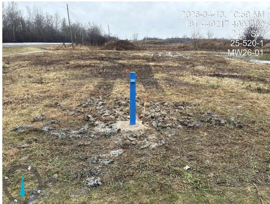
Photograph 1: Photograph of installed MW26-01.
