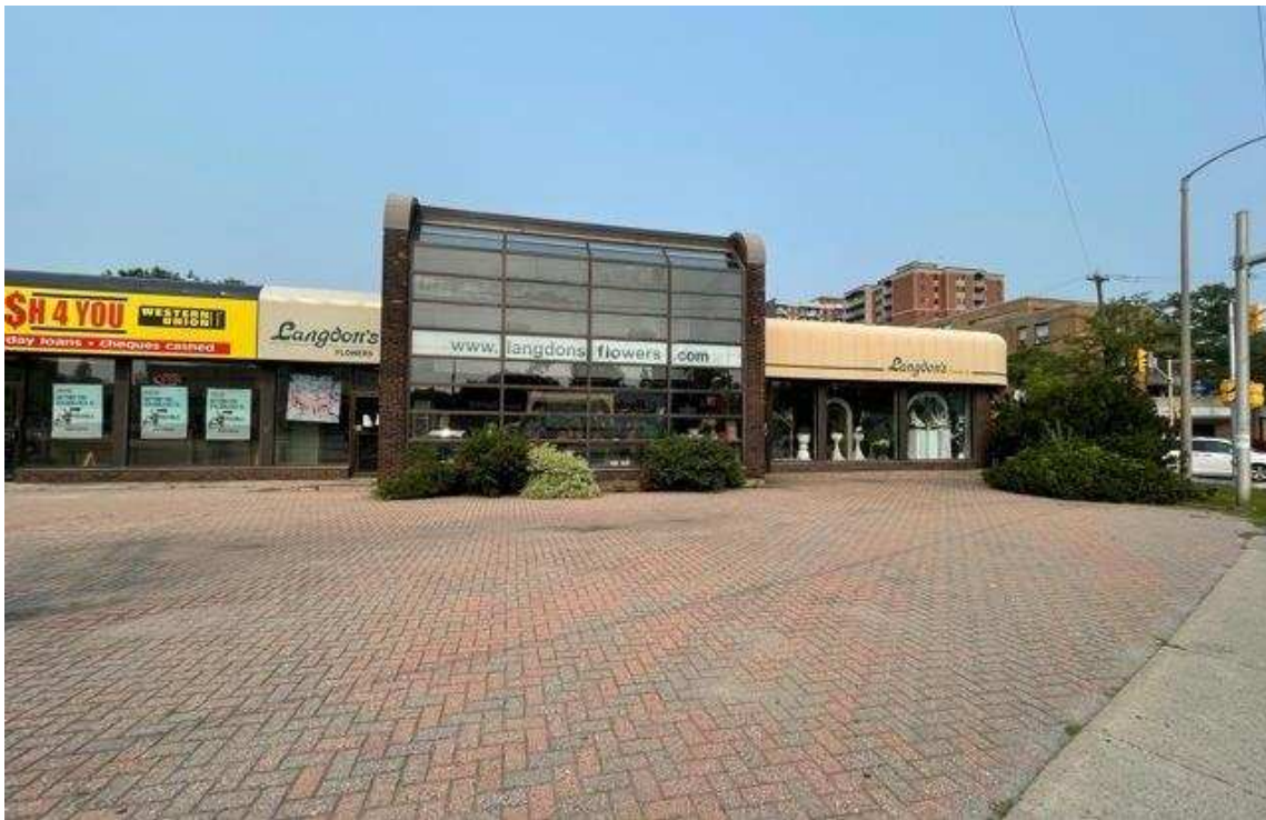
Photograph 2: View of the store fronts of the subject building. Photograph taken looking northwest.
