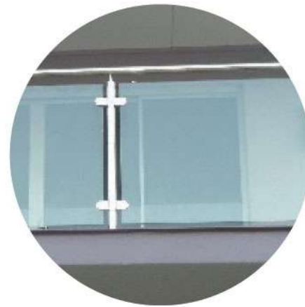
7. BALCONY METAL SIDING
