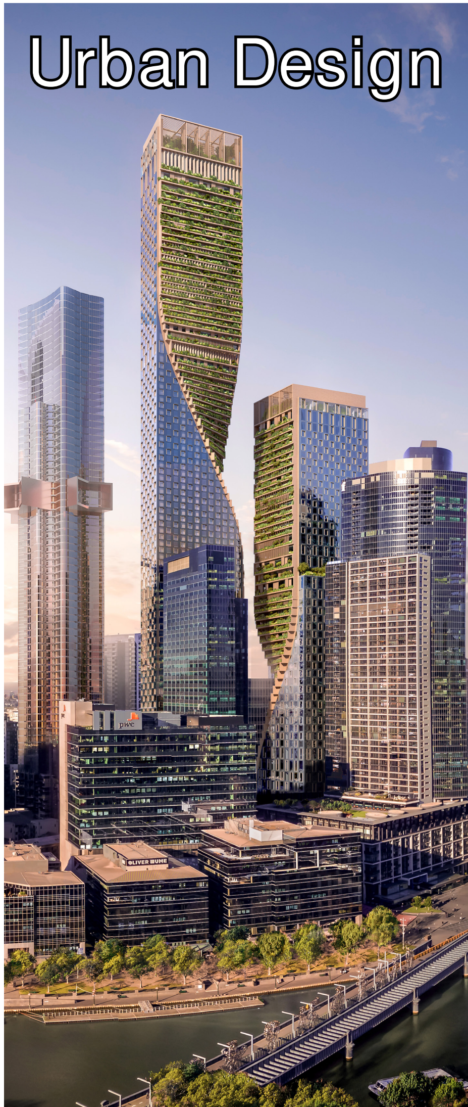
South Bank, Melbourne under construction
