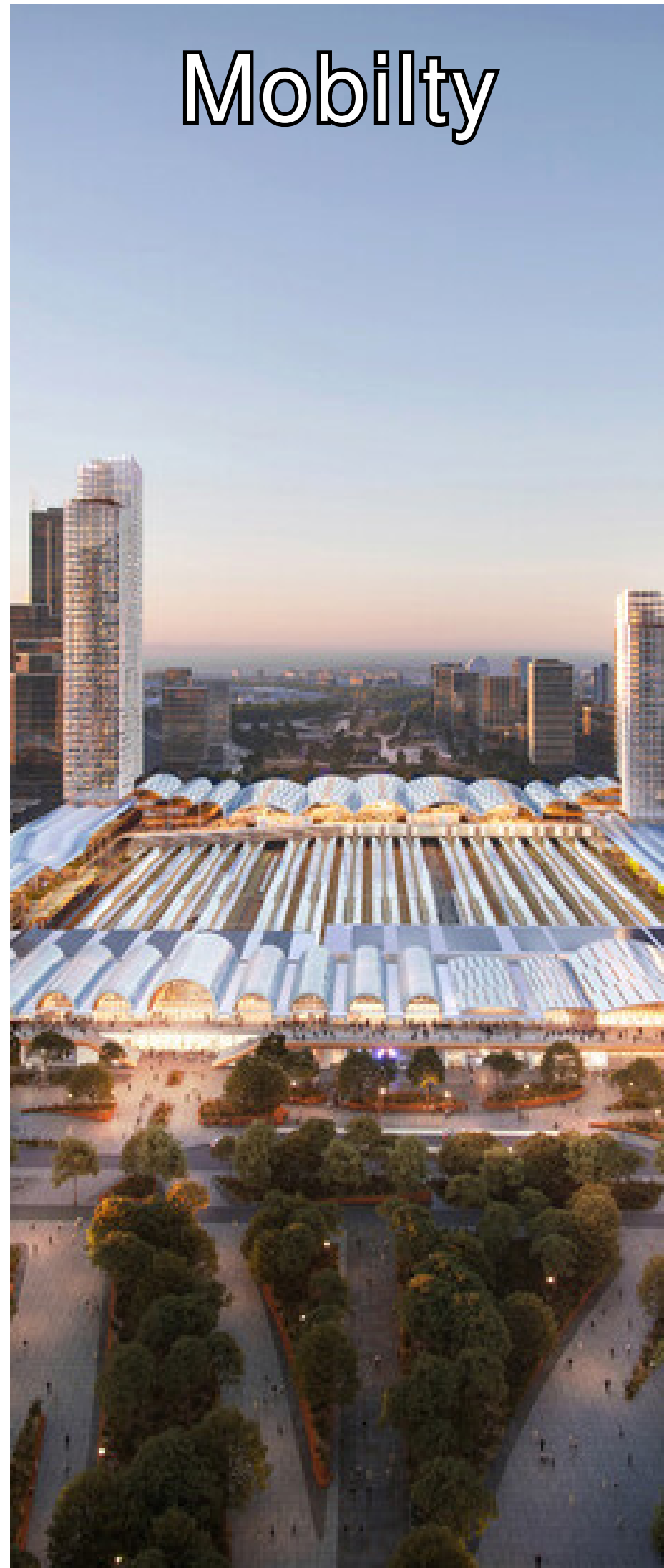
Chamartin Station, Madrid under construction
