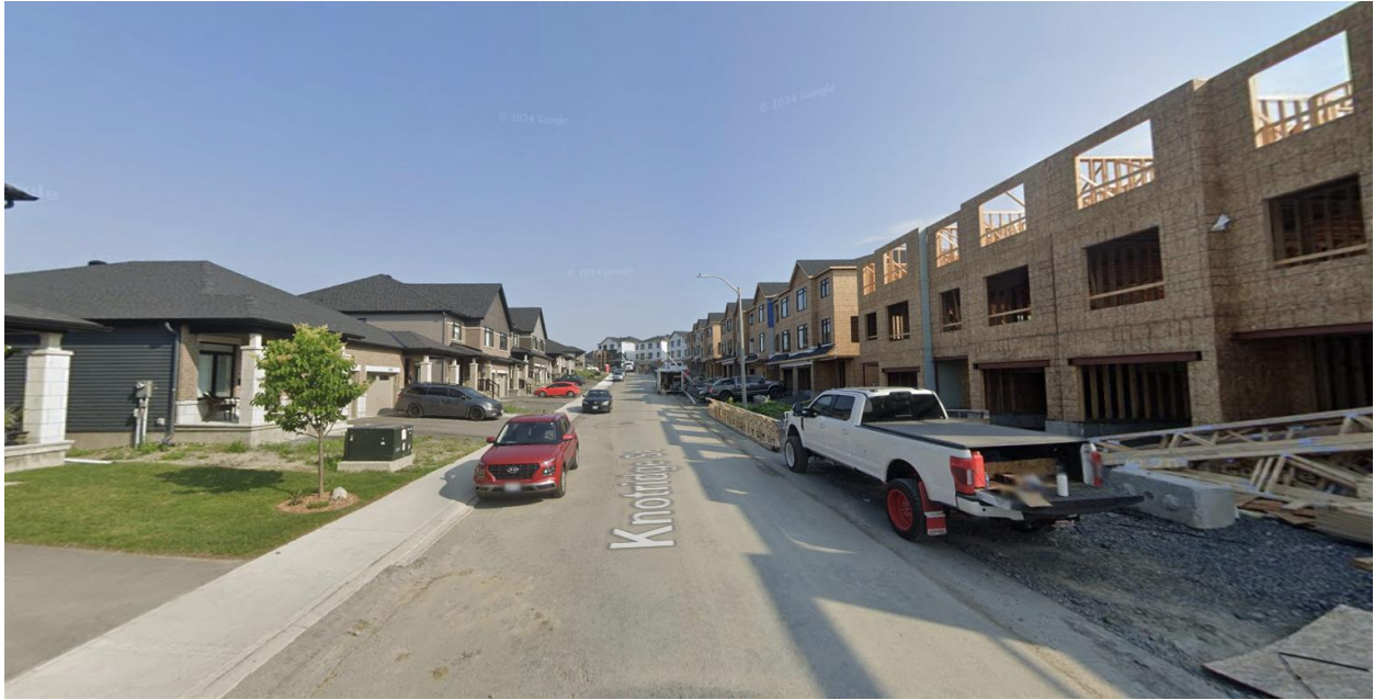
Figure 9: Detached and townhouse dwellings on Knotridge Street (looking north) (Google Streetview, July 2023).
