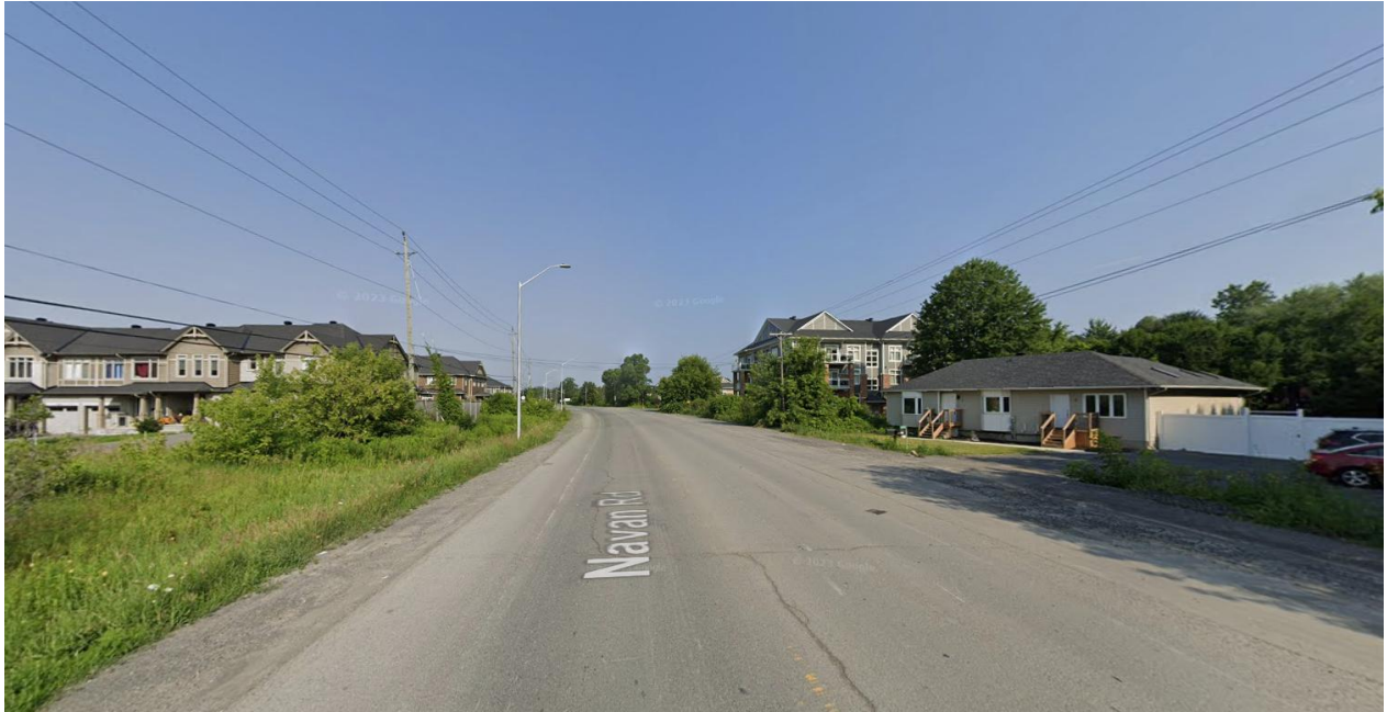
Figure 5 : Single detached and townhouse dwellings along Navan Road (looking north-west) (Google Streetview, July 2023).
