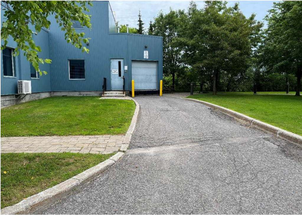
Photograph 1: Rear addition of the subject building, looking at the shipping and receiving dock.
