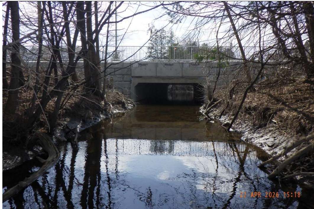
Photo 12: Reach FC-1a Findlay Creek, Ottawa, Ontario Photo Direction: Upstream
