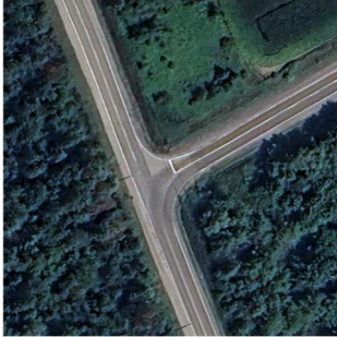
Leitrim Road (North Leg) at Ramsayville Road
