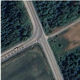
Leitrim Road (South Leg) at Ramsayville Road
