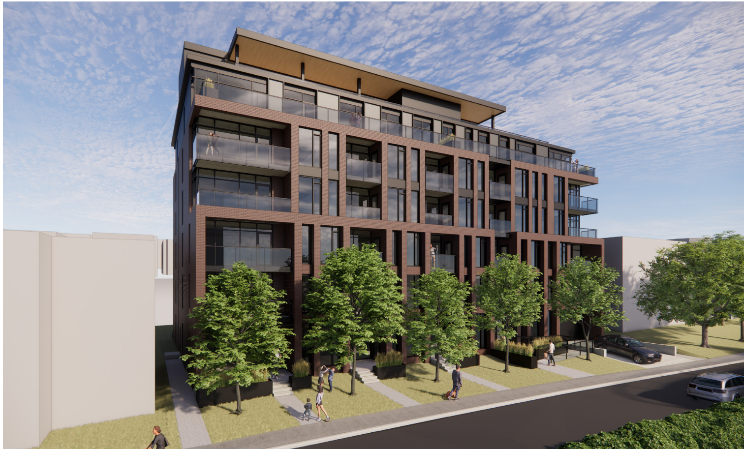
View of West Facade from Echo Drive
