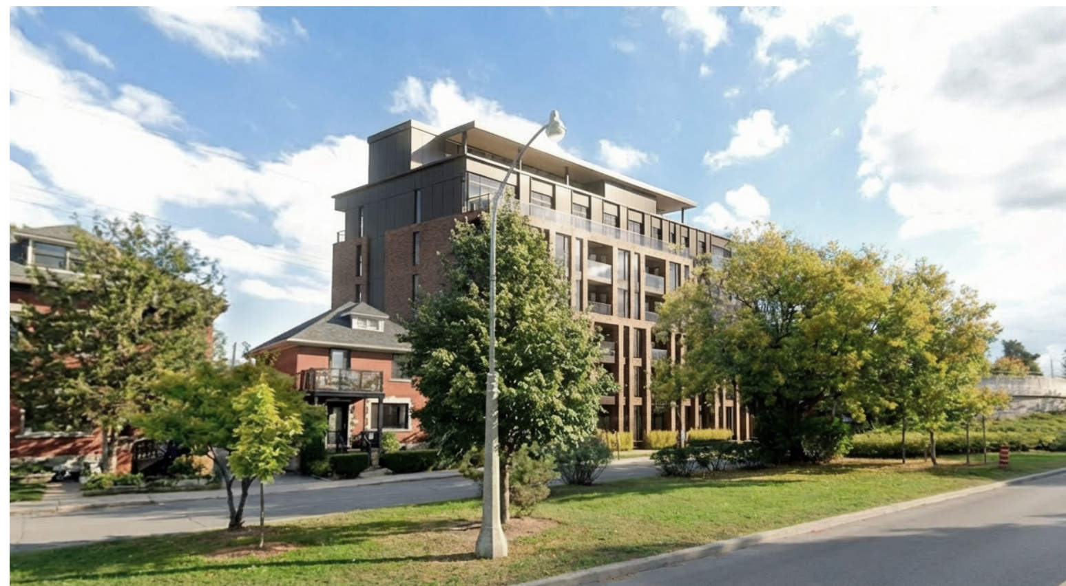
View From Colonel By Drive Looking South-East
