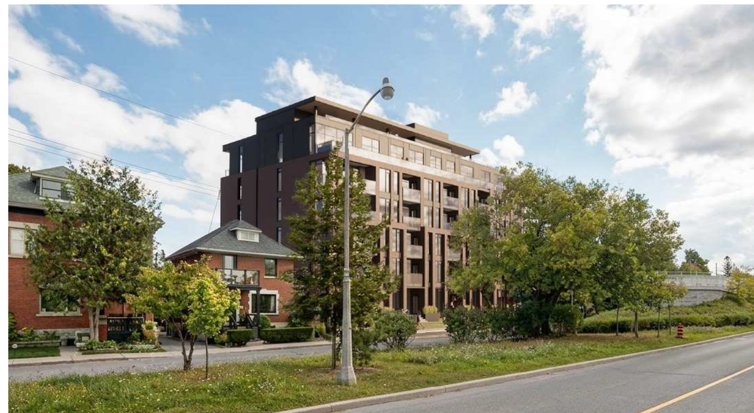
View From Colonel By Drive Looking South-East
