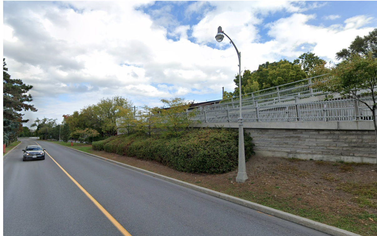
3. Looking North along Colonel By Drive
