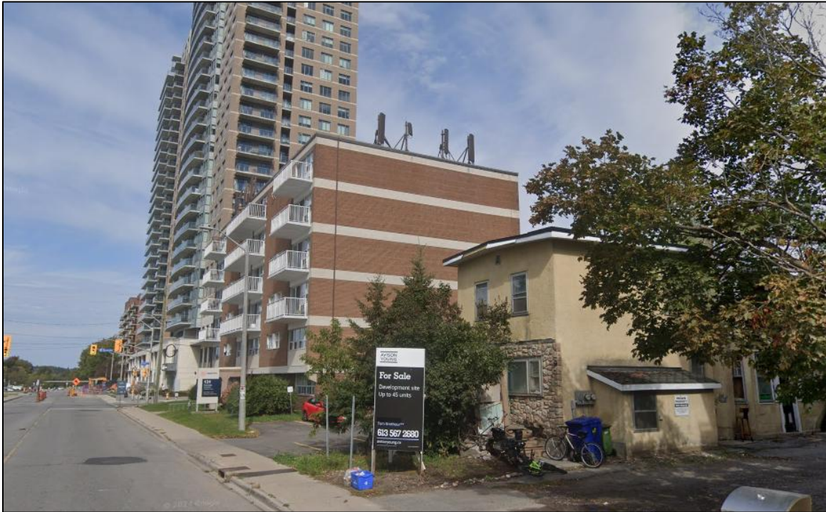
Figure 2 Views of the existing apartment buildings at 131 and 139 Parkdale Ave facing northeast from Parkdale Ave.
