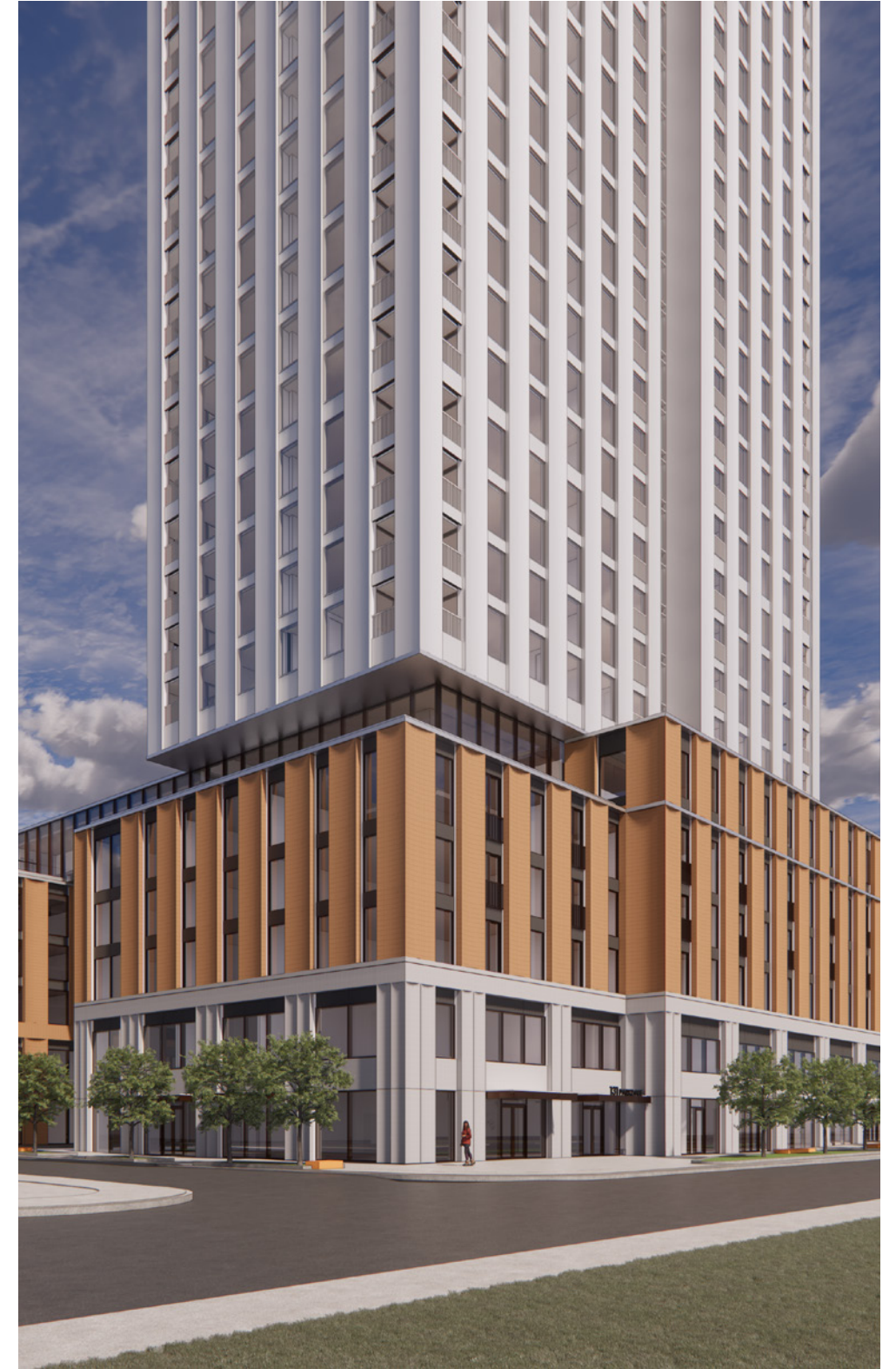
No Horizontal Datum at Tower Double Scallop Panel at Ground Floor
