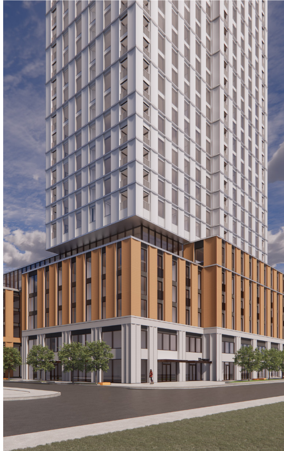
Horizontal Datum at Tower Double Scallop Panel at Ground Floor
