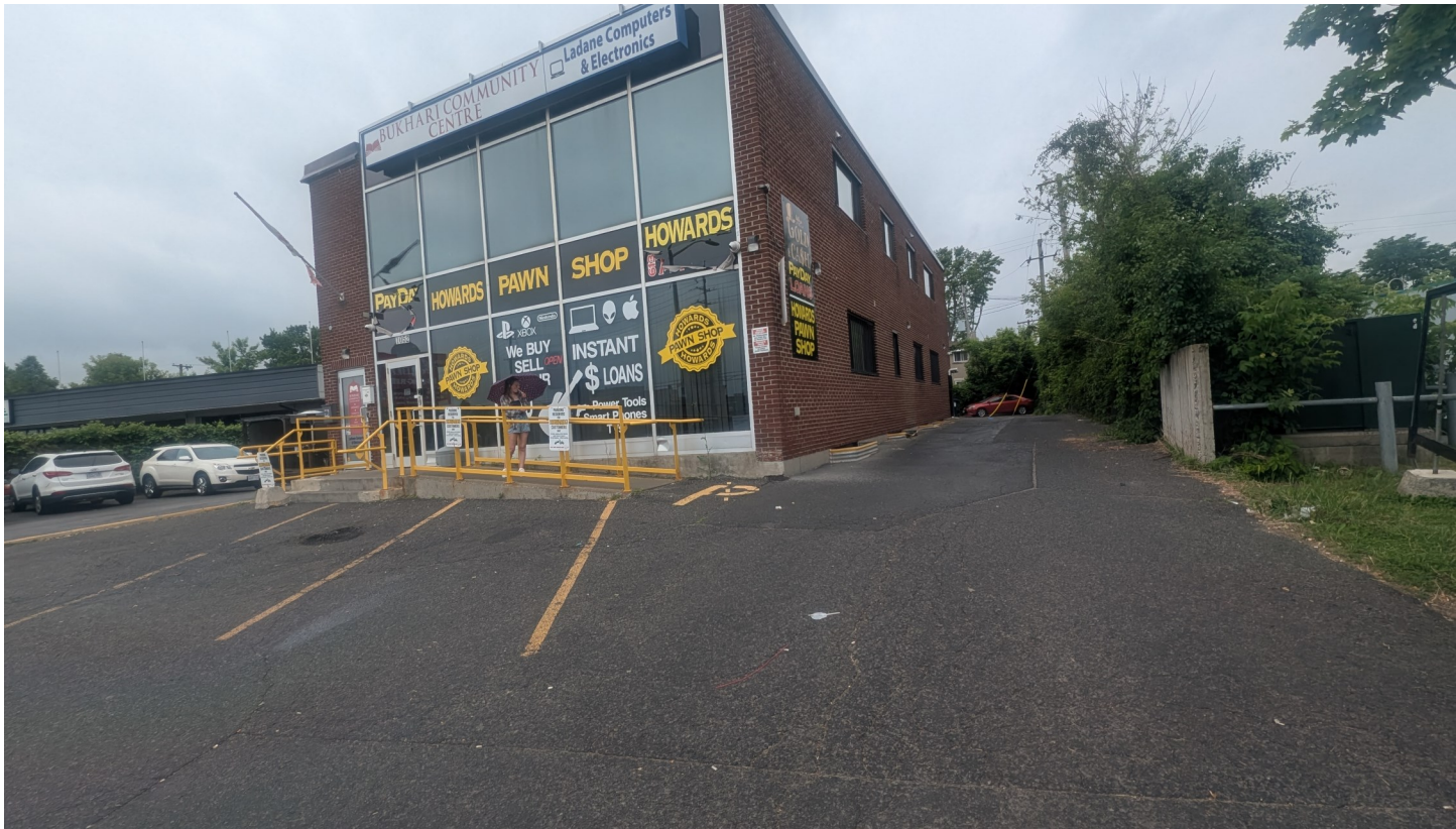
Photo 2 - Looking west towards the east building line of structure at 1052 St. Laurent Boulevard.
