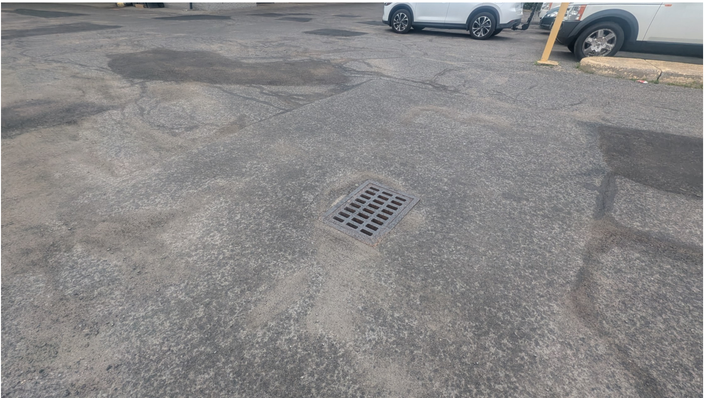
Photo 14 - Looking north/northwest towards the catch basin at 1064 St. Laurent Boulevard.
