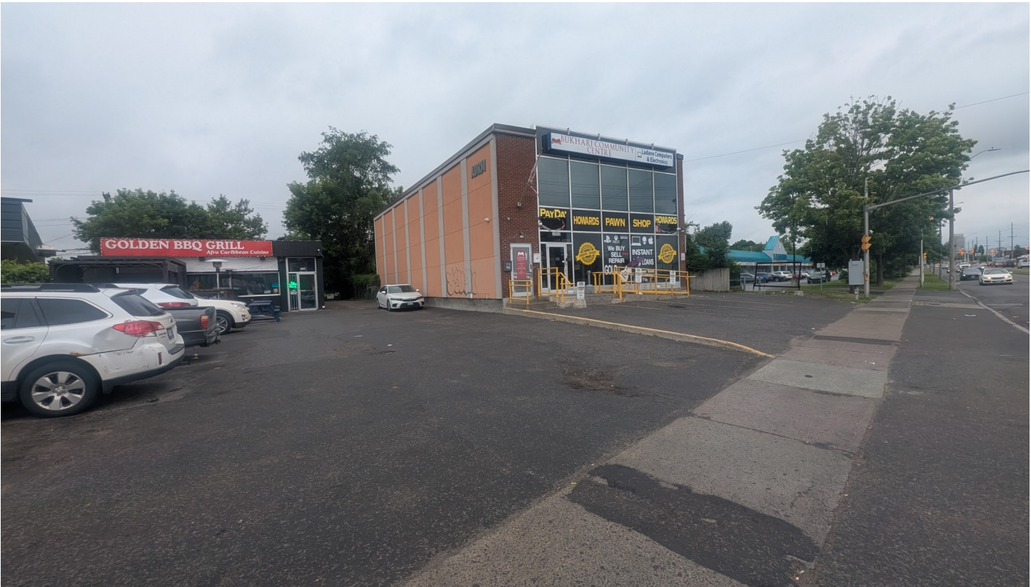
Photo 1 - Looking northwest towards the structure at 1052 St. Laurent Boulevard.
