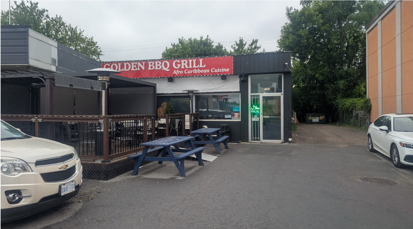
Photo 7 - Looking west towards the east building line of 1060 St. Laurent Boulevard.
