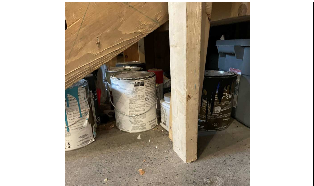
Photo 012 View of paint stored inside Mino'Weesini located at 5 Hamilton Avenue North (the Phase One Property) (facing east).
