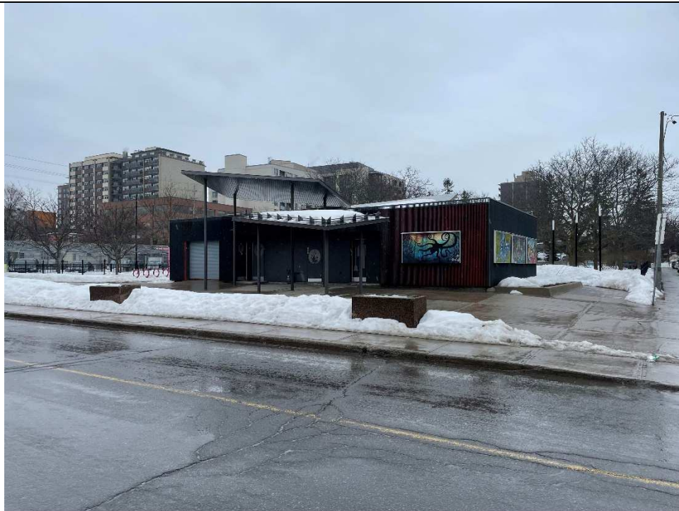
Photo 020 View of Parkdale Market/Parkdale Park directly south of the Phase One Property (facing southeast).
