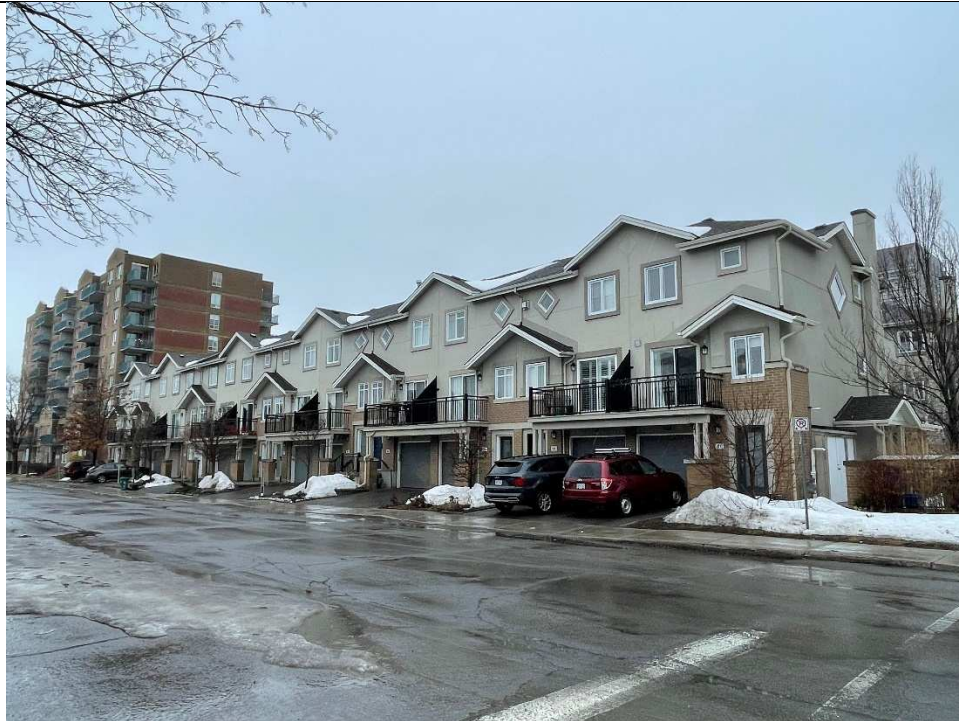
Photo 019 View of townhouses and an apartment building directly northwest of the Phase One Property (northwest).
