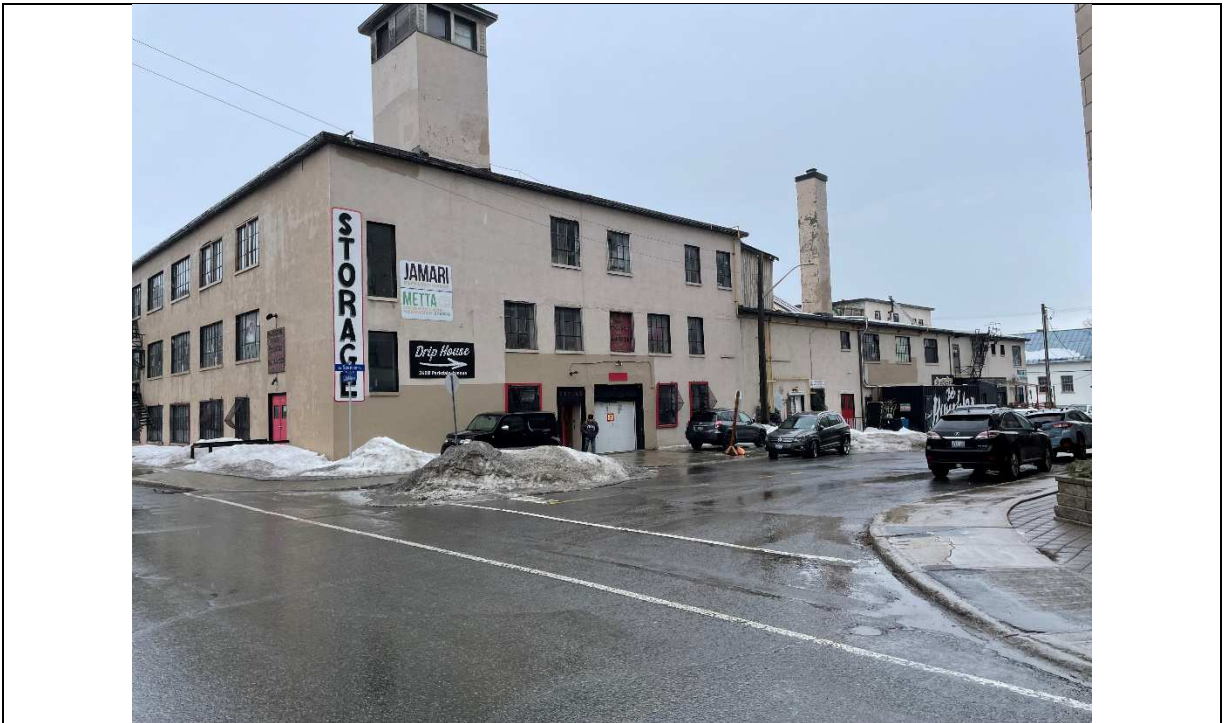
Photo 017 View of the northeast corner and northern portion of the Phase One Property (facing southwest).
