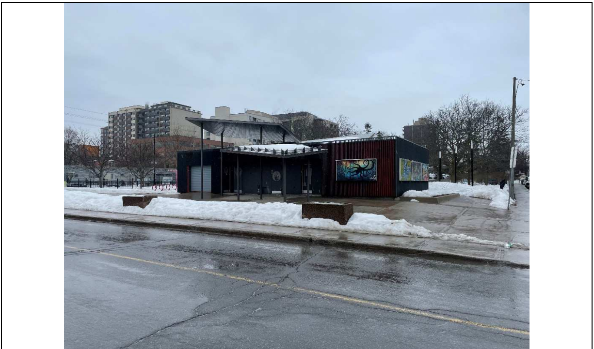
Photo 020 View of Parkdale Market/Parkdale Park directly south of the Phase One Property (facing southeast).
