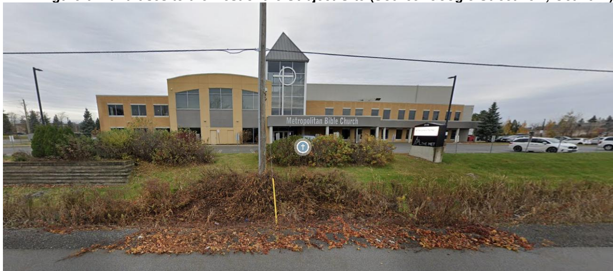
Figure 6: Land uses to the west of the Subject Site (Source: Google Streetview, Oct 2024)
