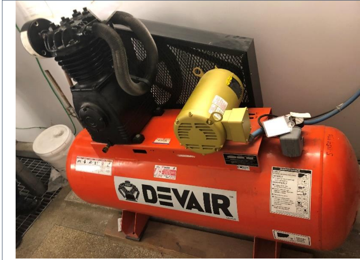
Picture 5 – Air Compressor Within 2 nd Floor Mechanical Room of Office Building
