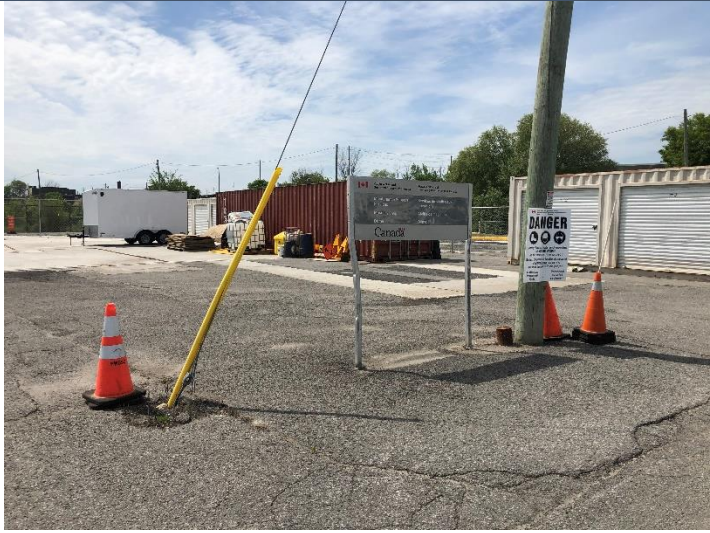
Picture 13 – Public Works Yard (facing southwest)
