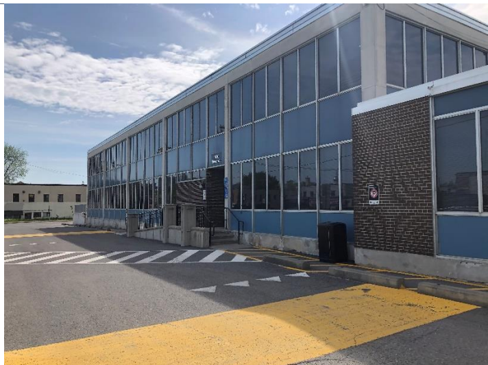
Picture 1 – Office Building on RSC Property (facing east)
