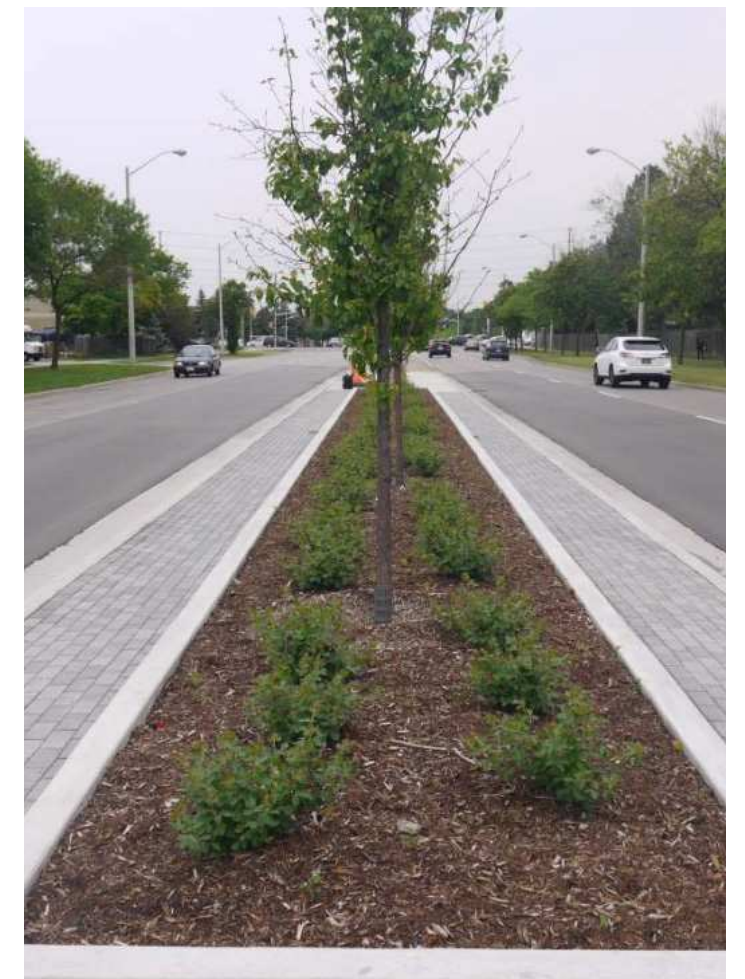
Figure 125: Stormwater tree trenches in Mississauga, ON. Source: CVC
