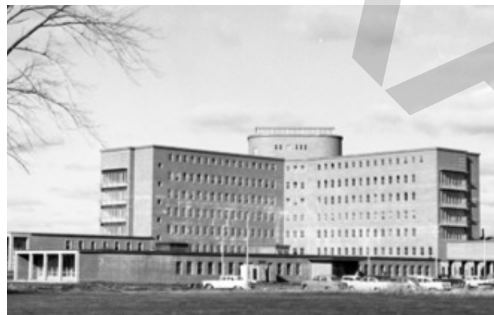
Figure 88: Tilley Building. Source: CLC
