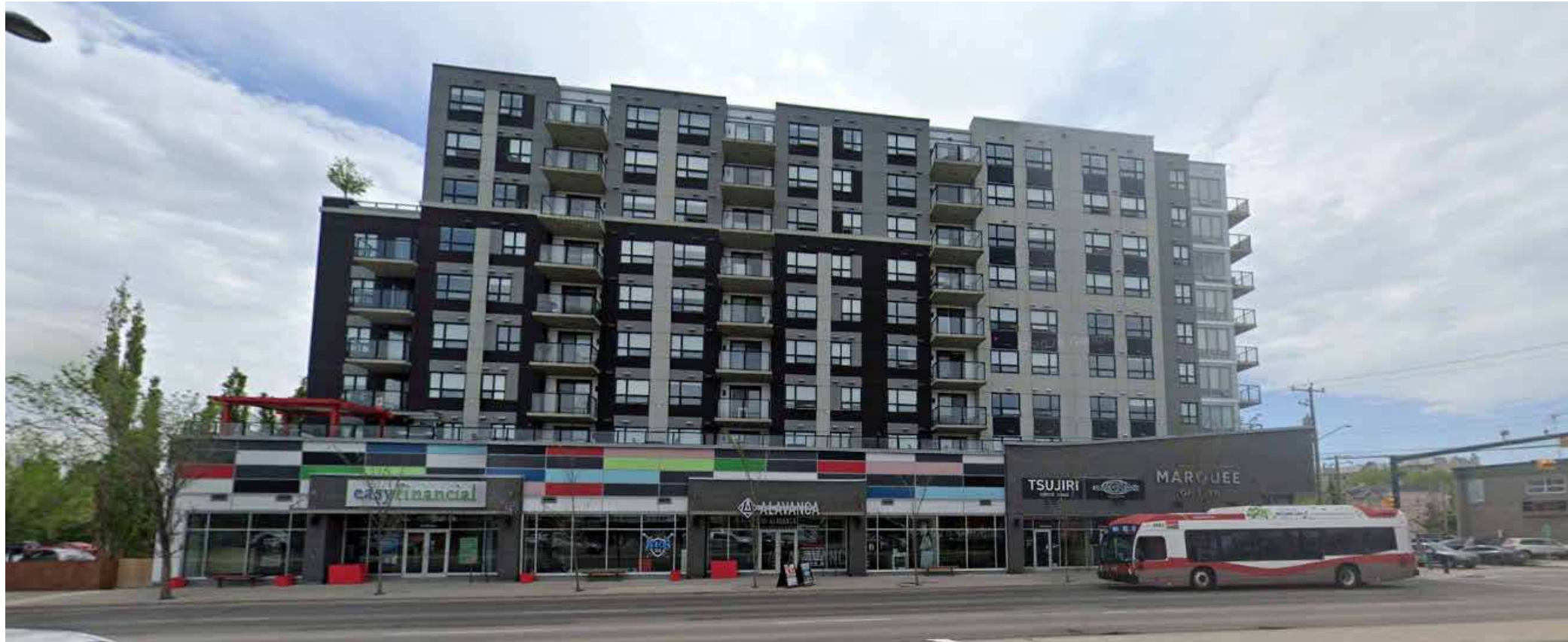
SITE PHOTO 4 - 16 AVENUE , LOOKING SOUTH
