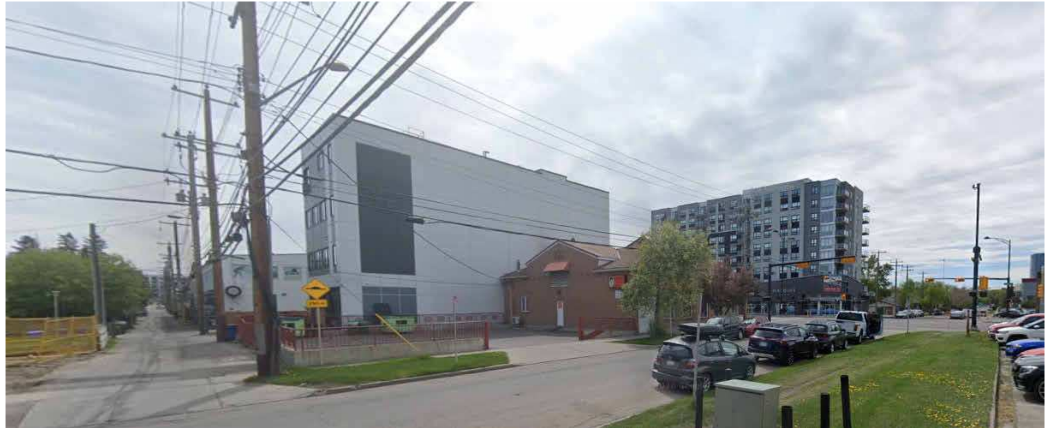
SITE PHOTO 3 - 1 STREET NE , LOOKING SOUTH WEST
