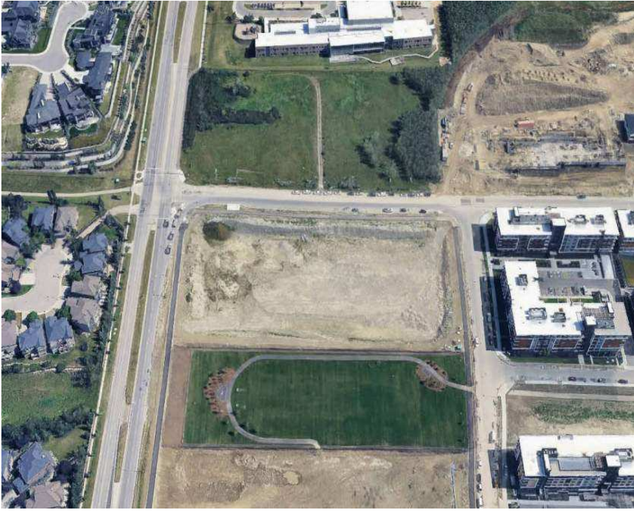
AERIAL VIEW WEST
