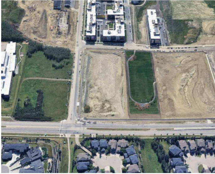
AERIAL VIEW NORTH
