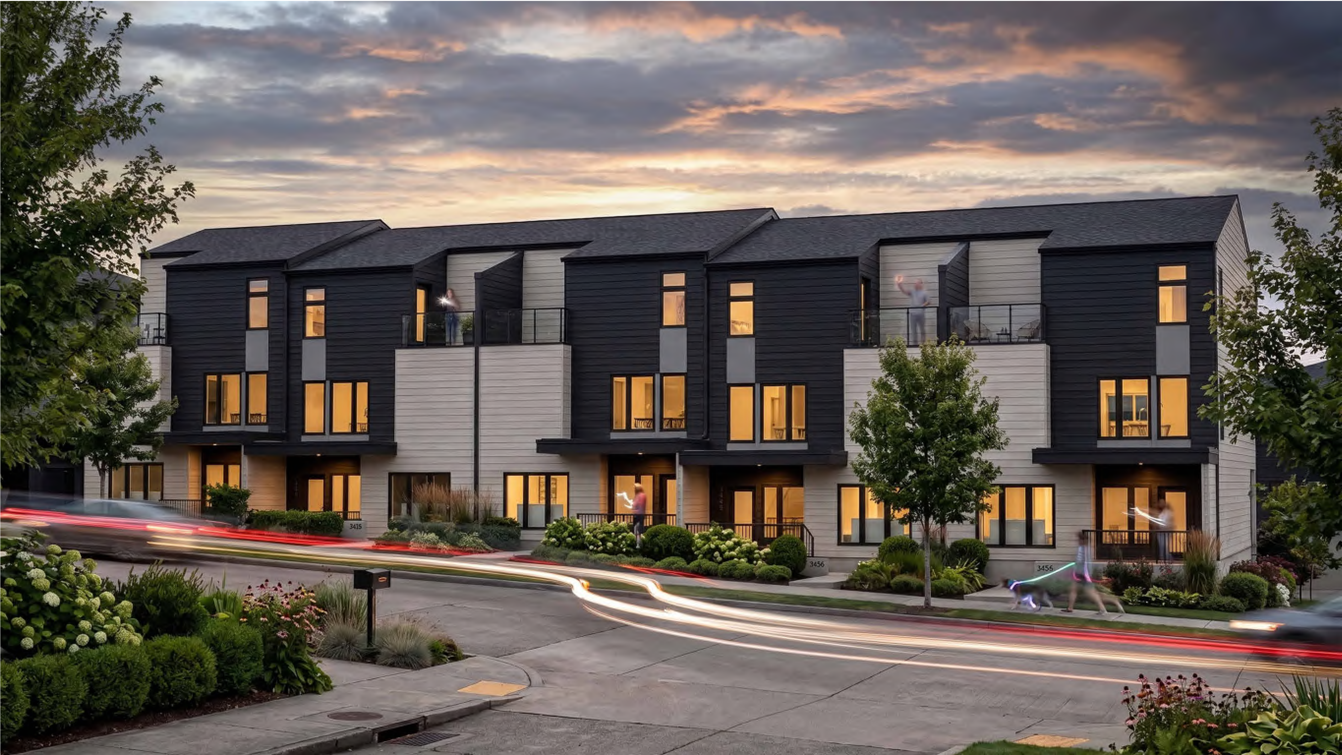
Building - B07 - Front
