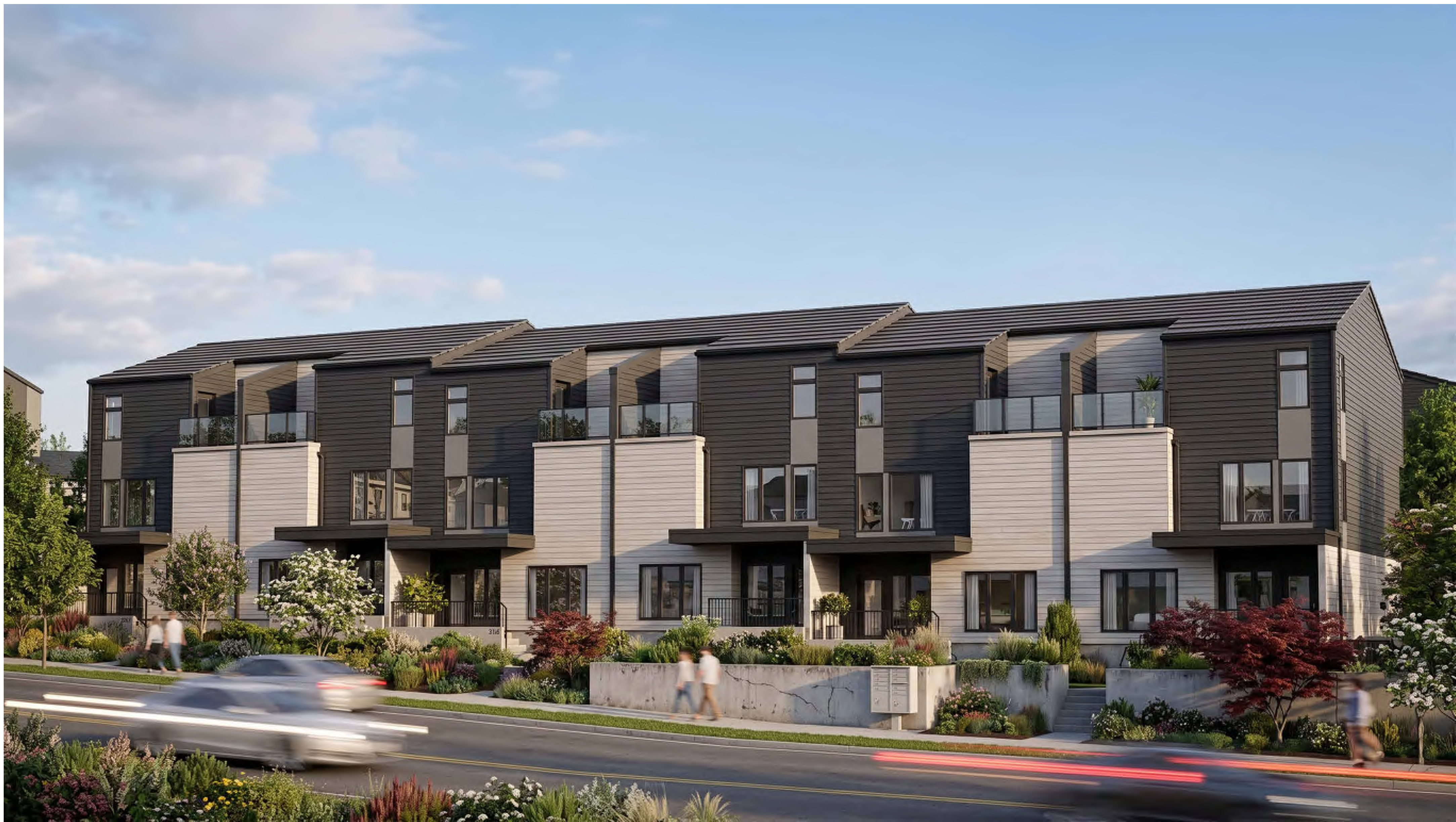
Building - B06 - Front
