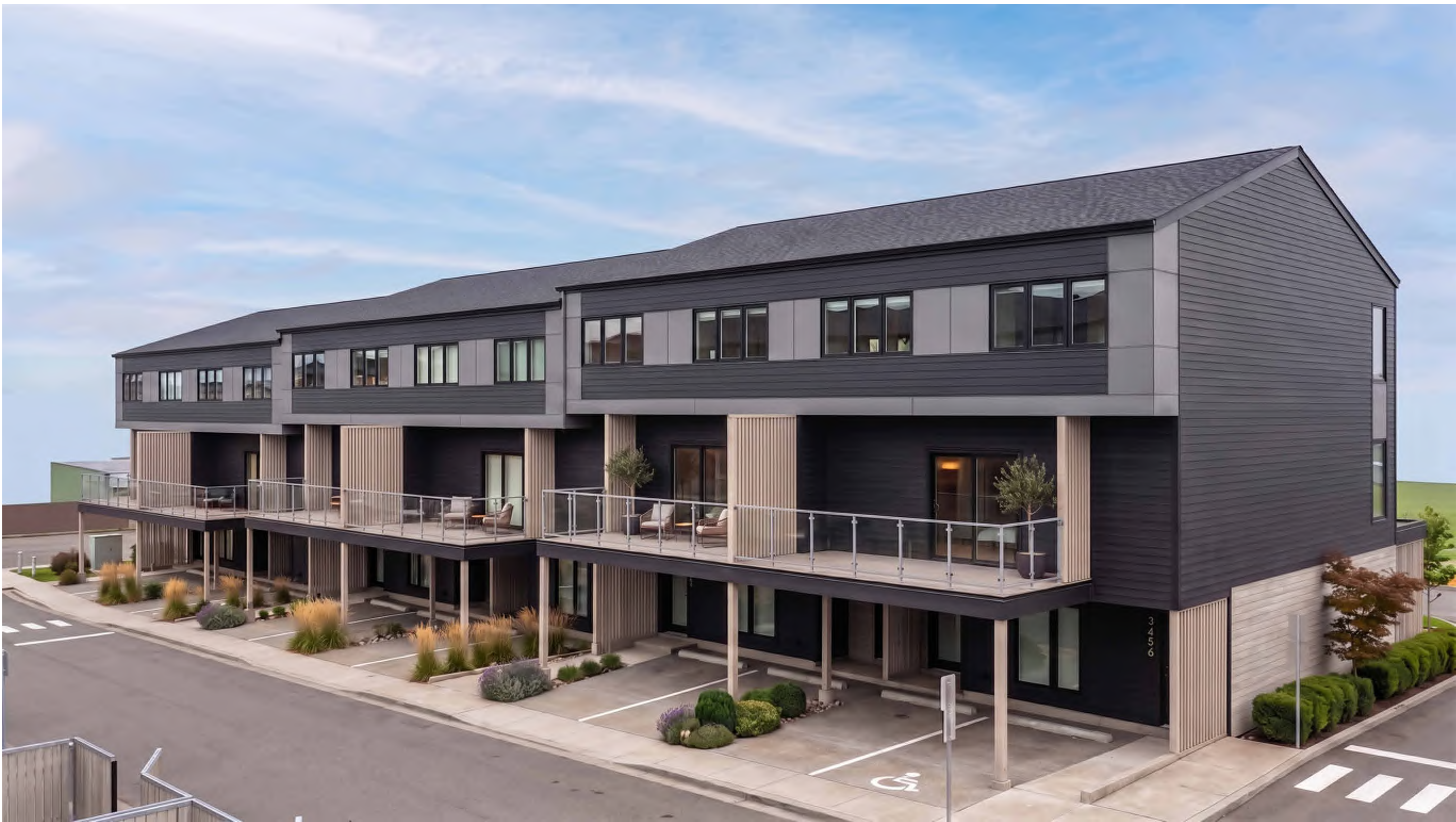
Building - B06 - Back
