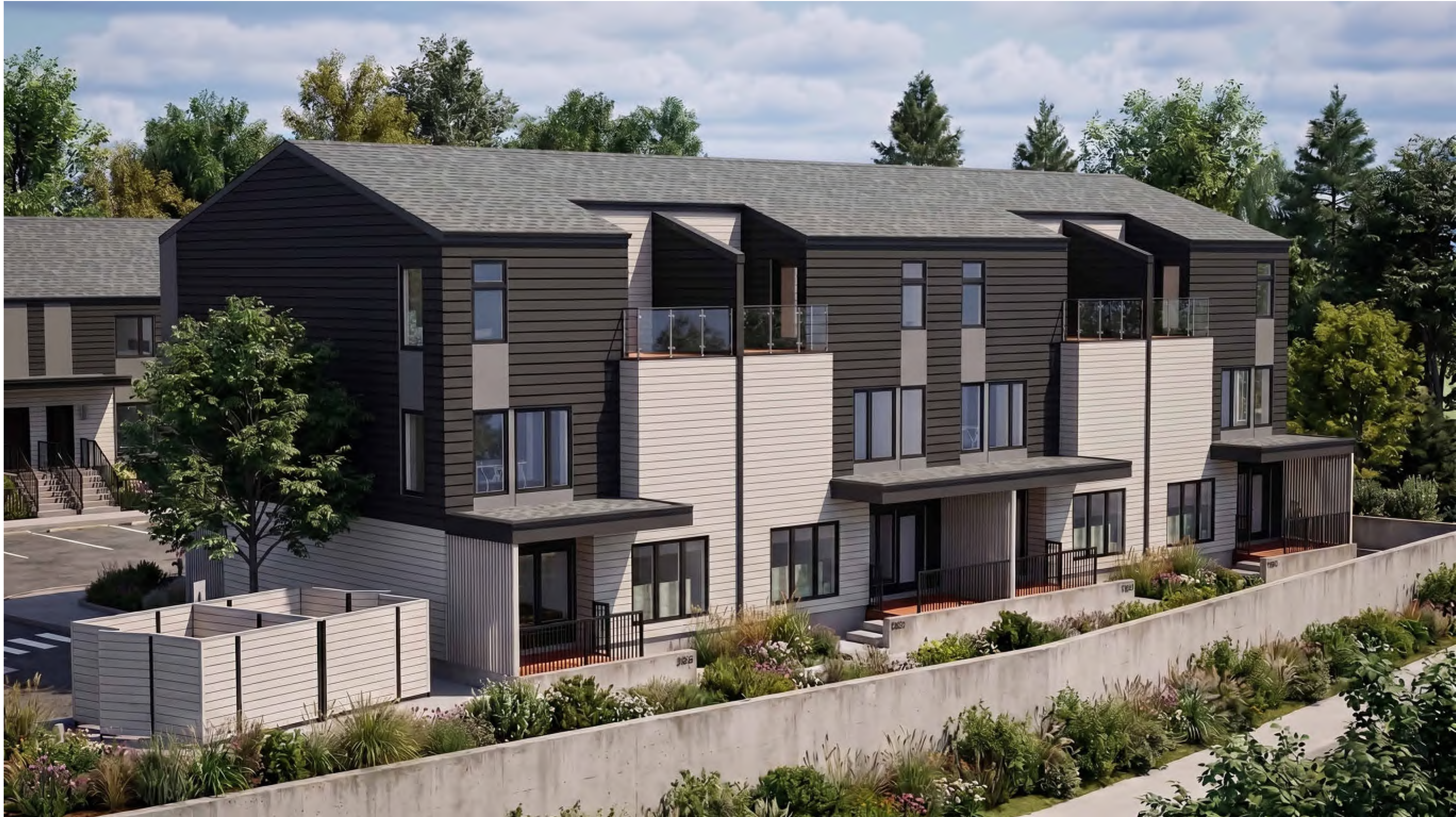
Building - B05 - Front
