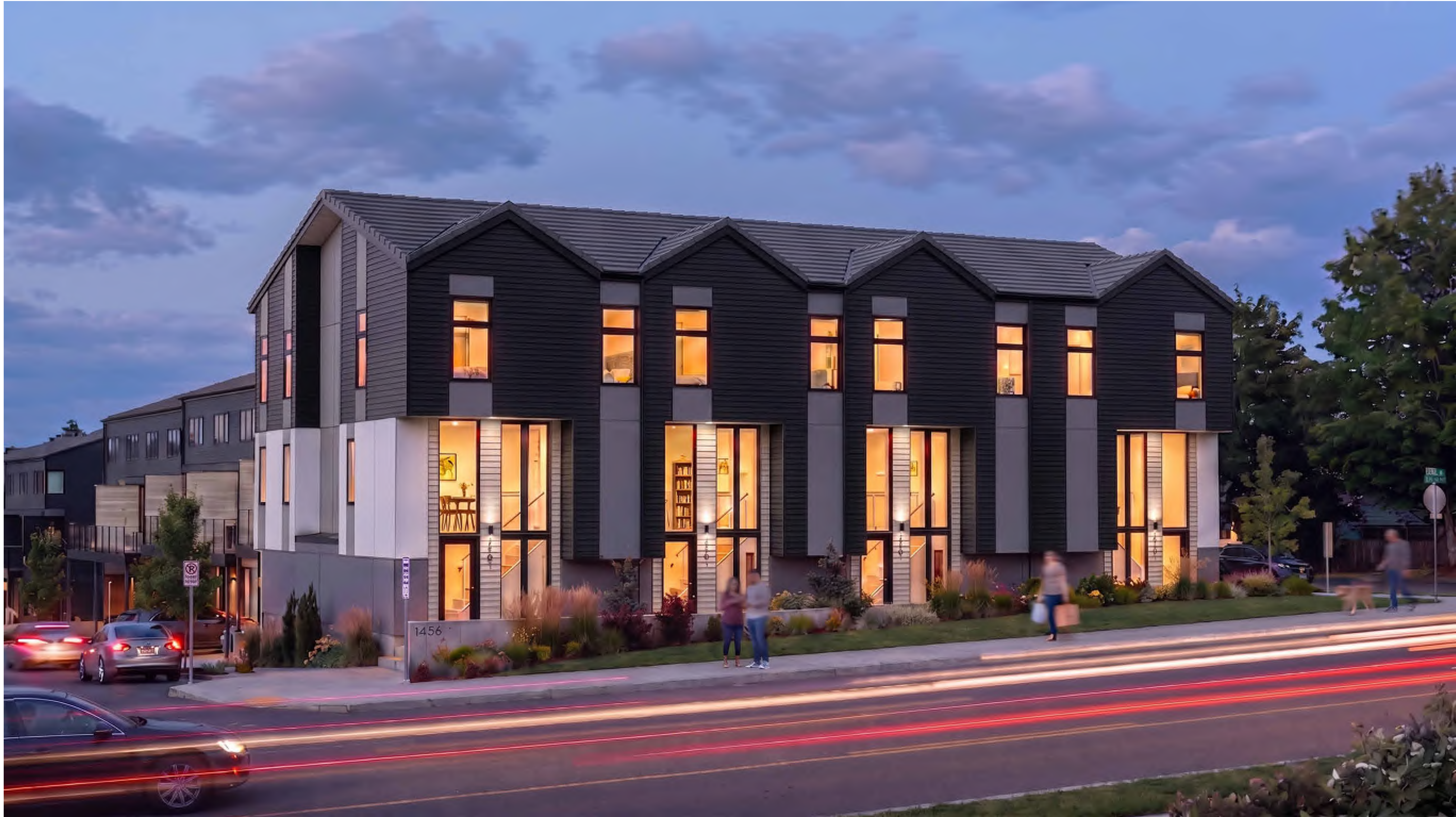
Building - B01 - Front
