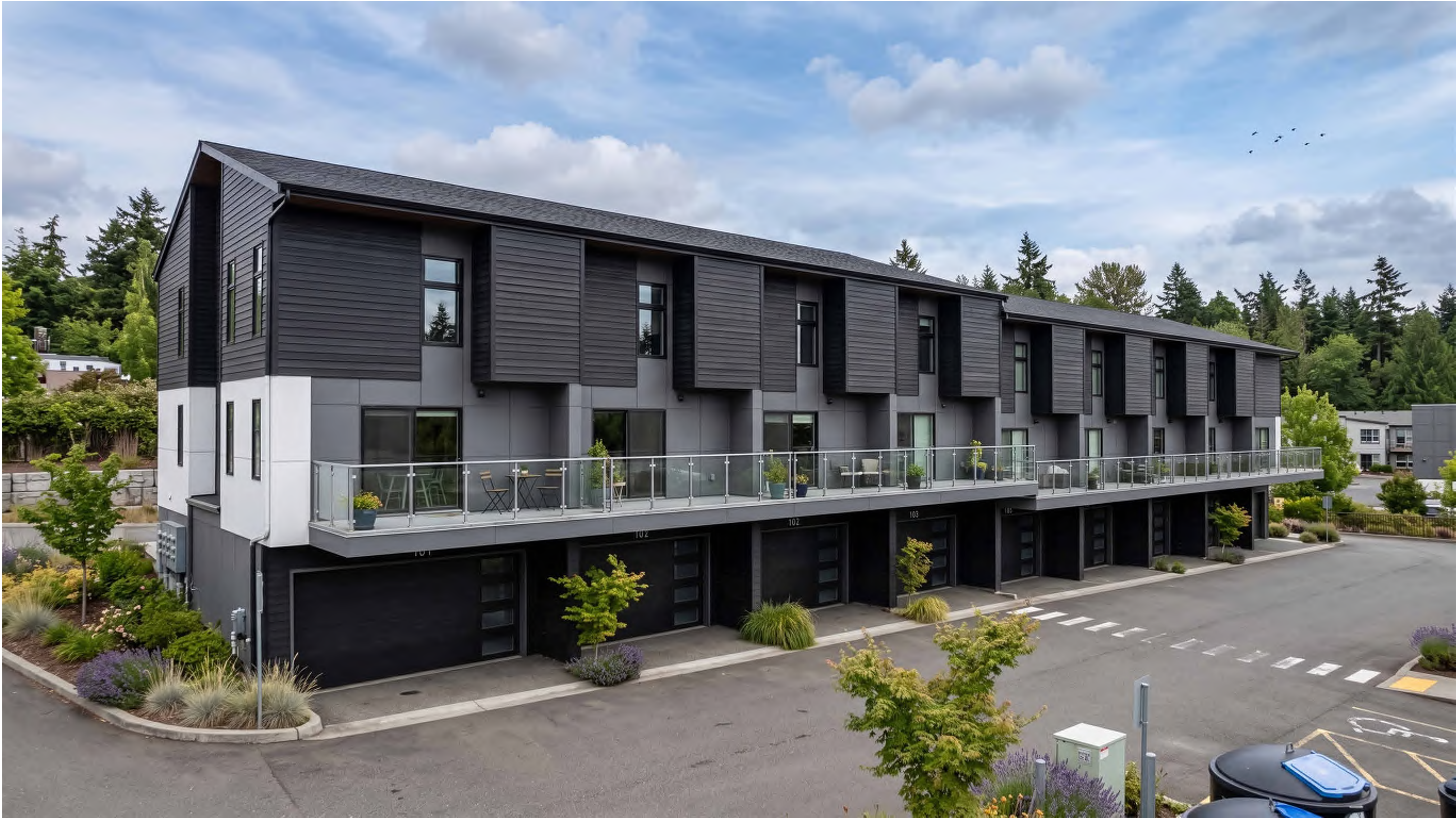
Building - B02 - Back
