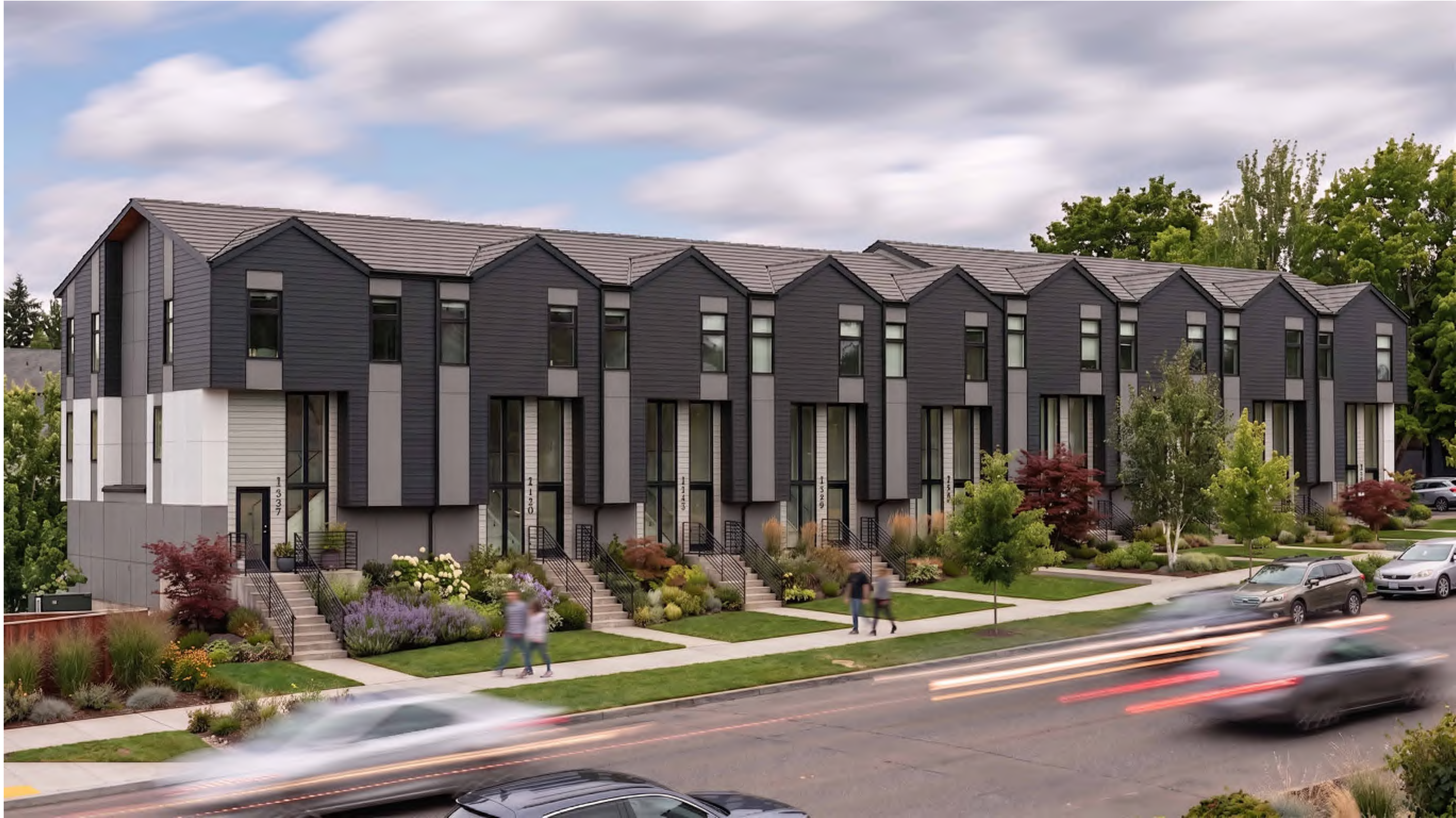
Building - B02 - Front
