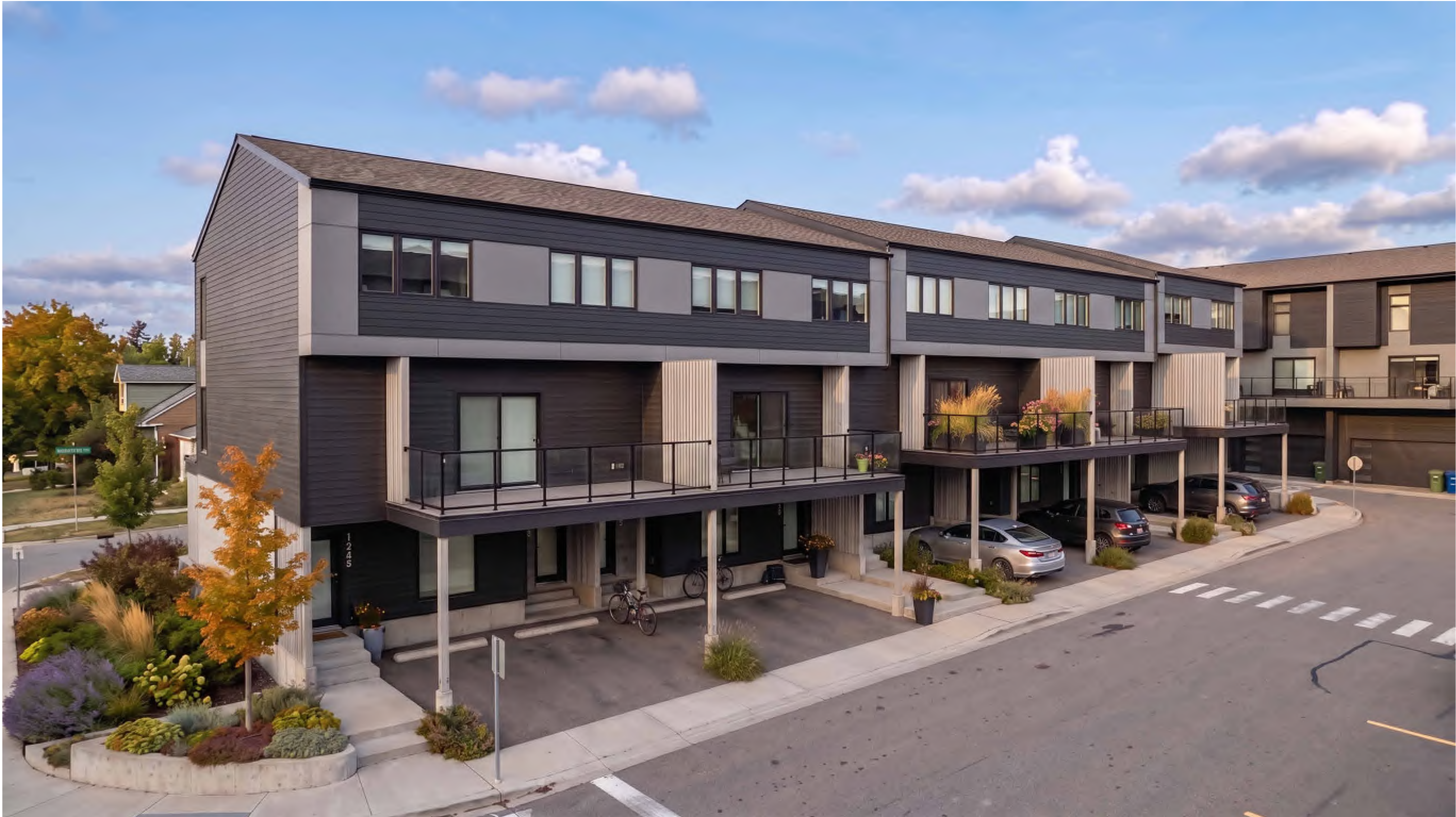
Building - B07 - Back
