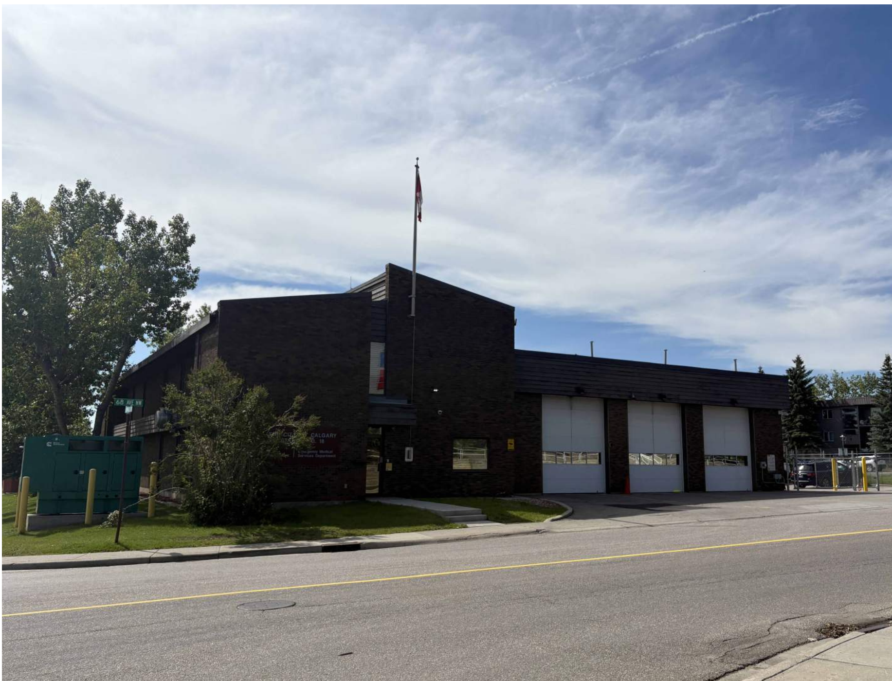
9 VIEW FROM NORTH CORNER OF SITE
