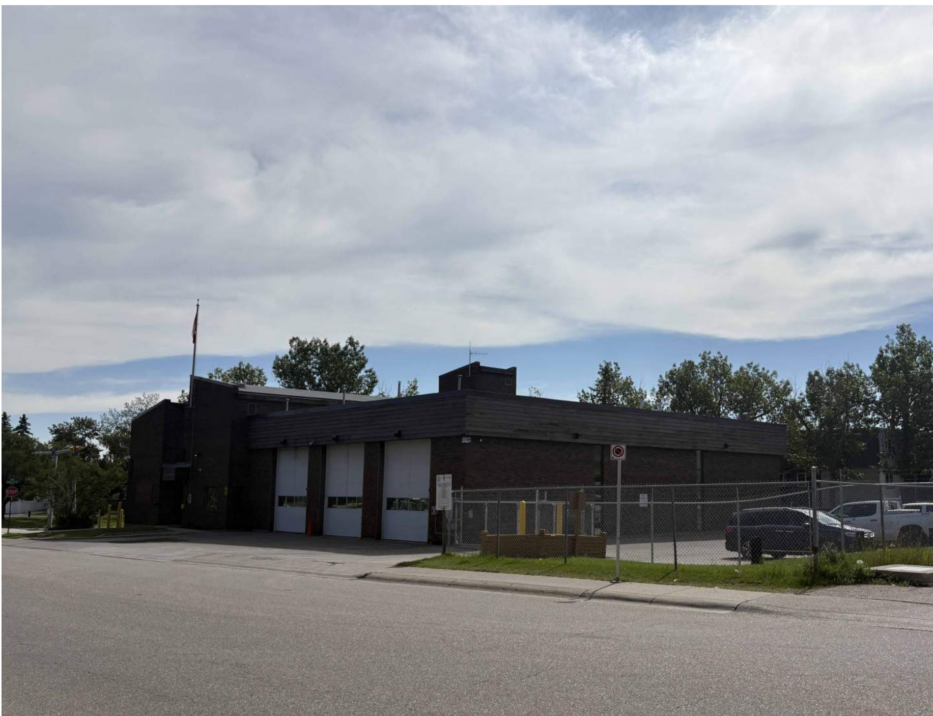
3 VIEW FROM WEST CORNER OF SITE
