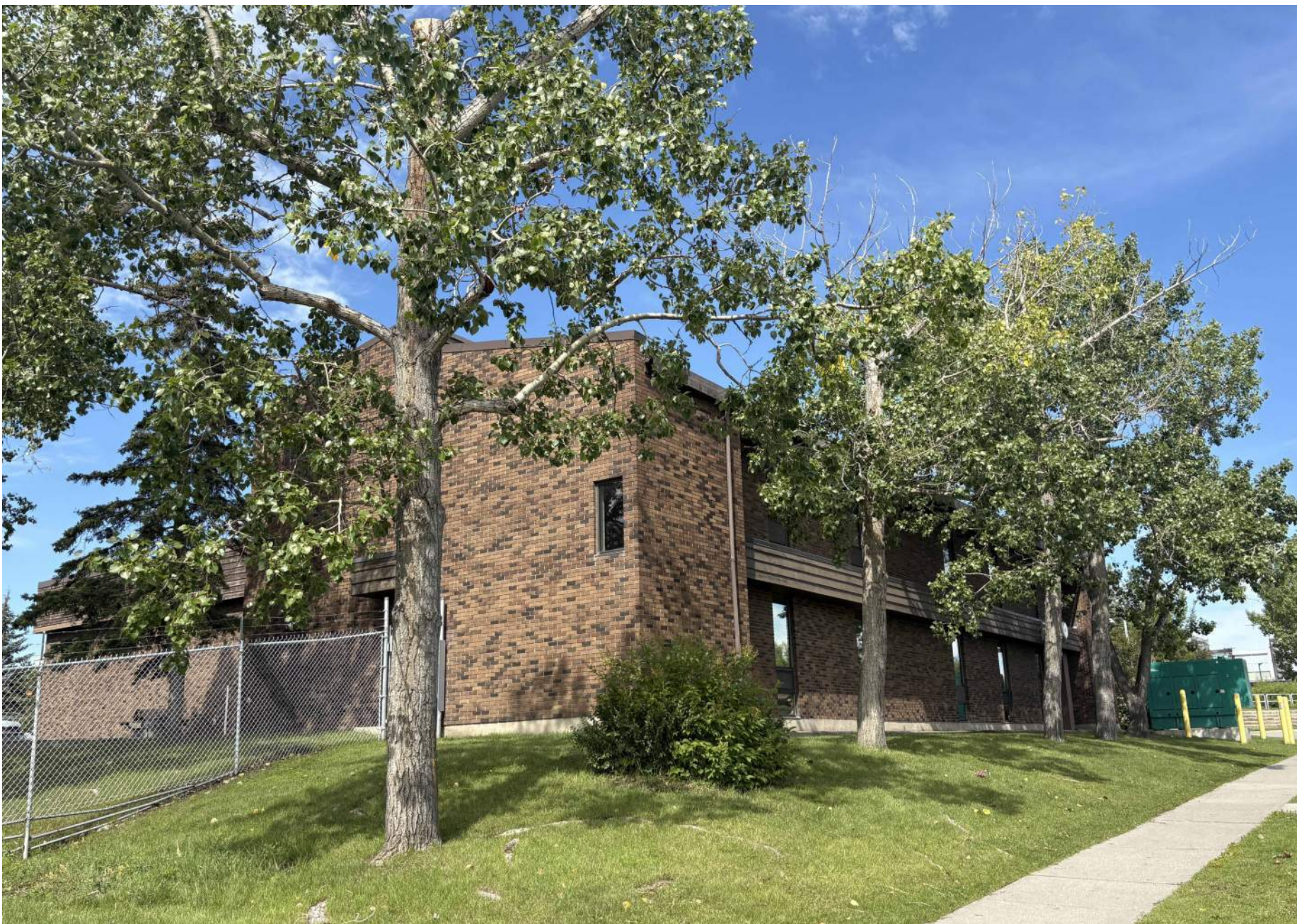
7 VIEW FROM EAST CORNER OF SITE
