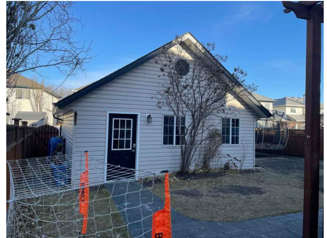
view of garage from ne corner of house
