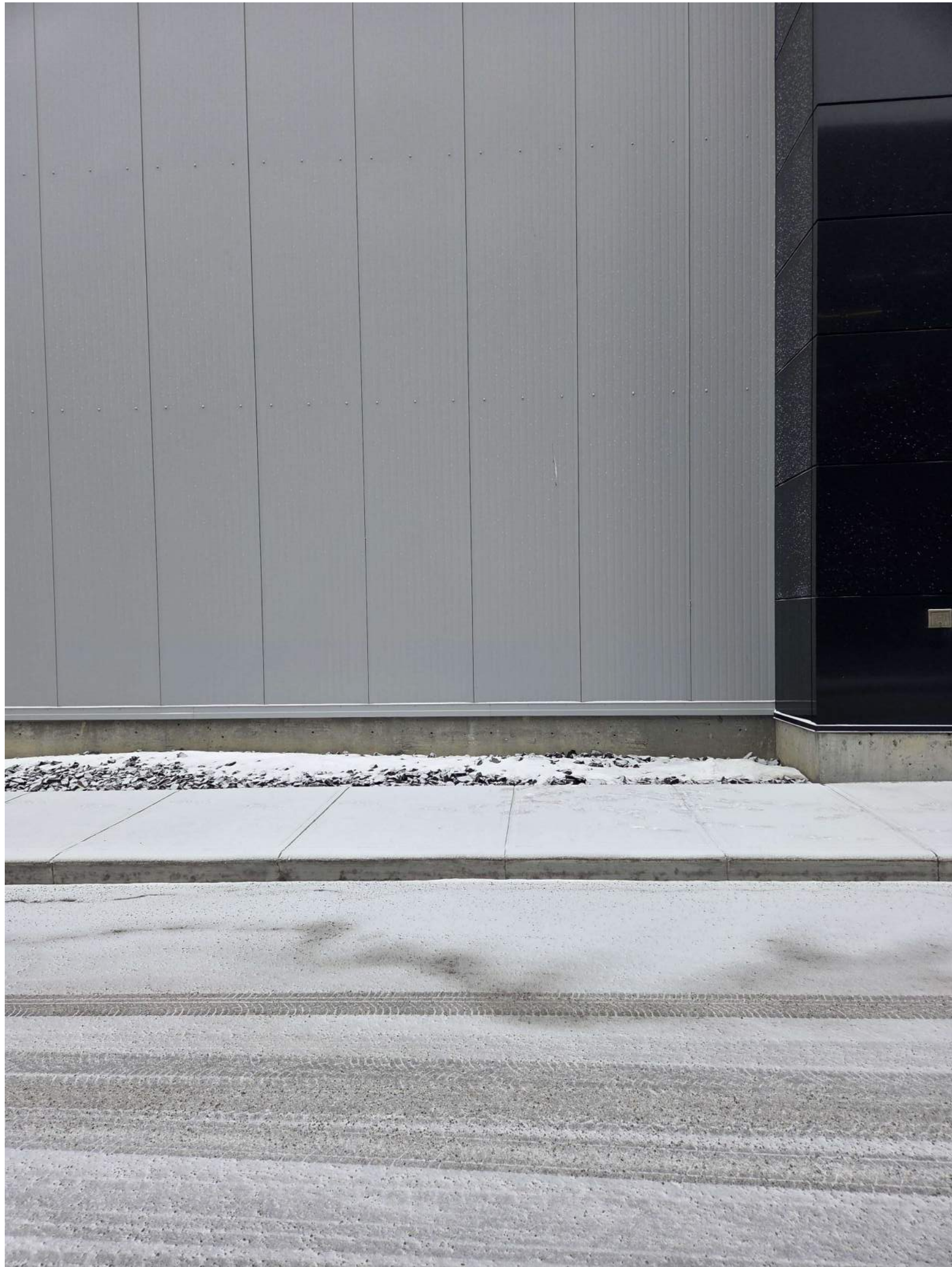
1 EXTERIOR PHOTO 1 DP2.00 1" = 20'-0"
