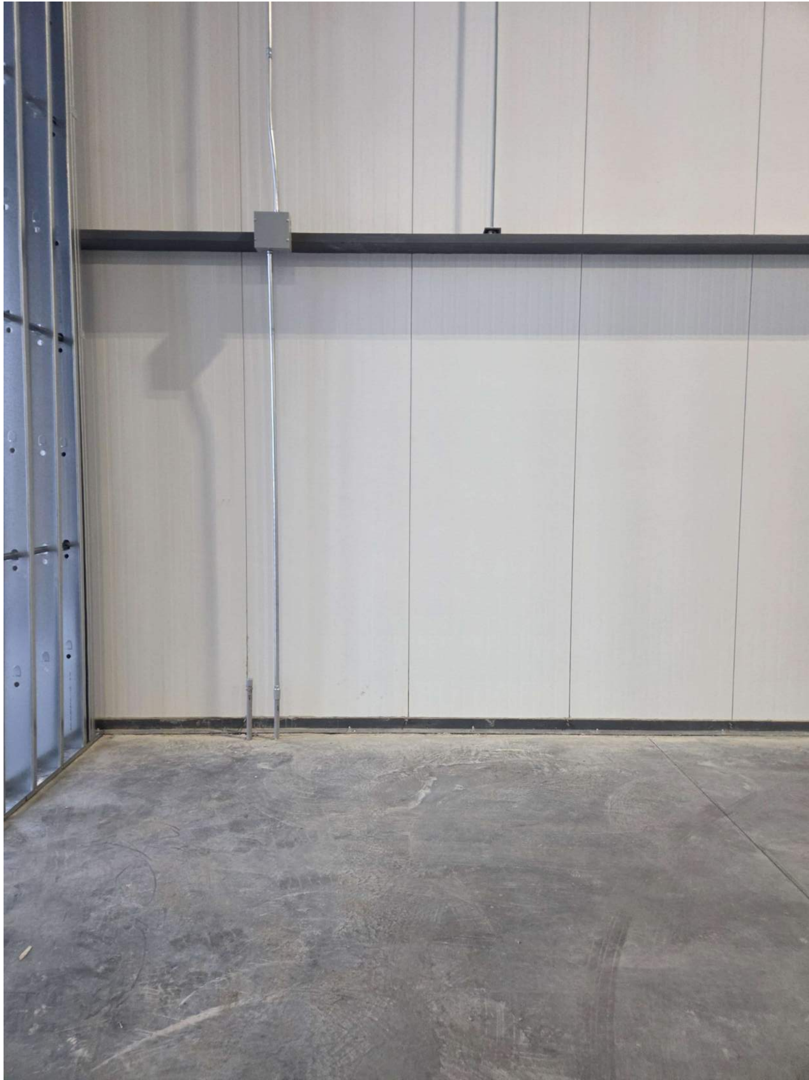
3 INTERIOR PHOTO 2 DP2.00 1" = 20'-0"
