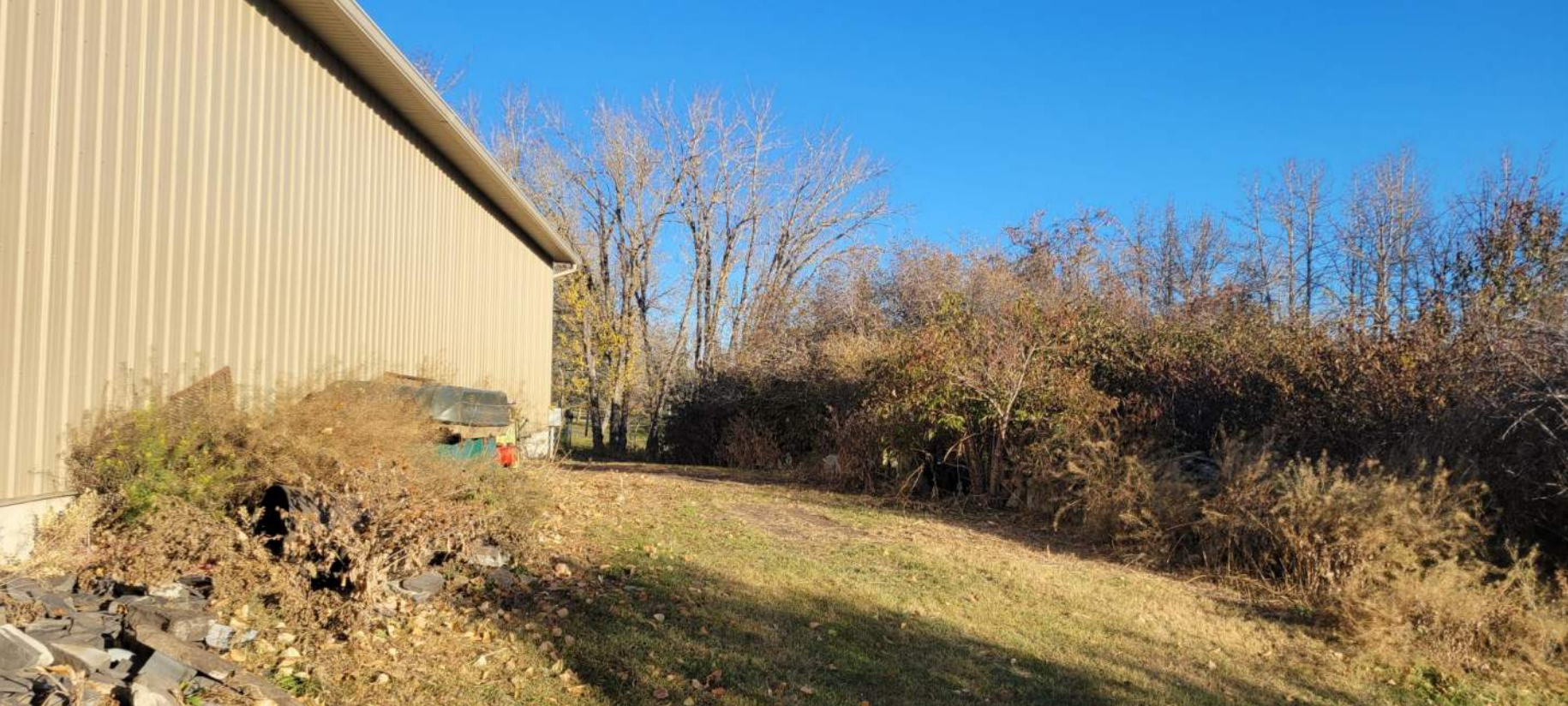
View from eastern edge of maintenance area looking north toward building site
