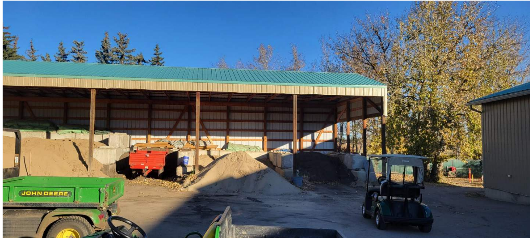
View from existing maintenance area parking looking north (site is to the right between the two buildings)
