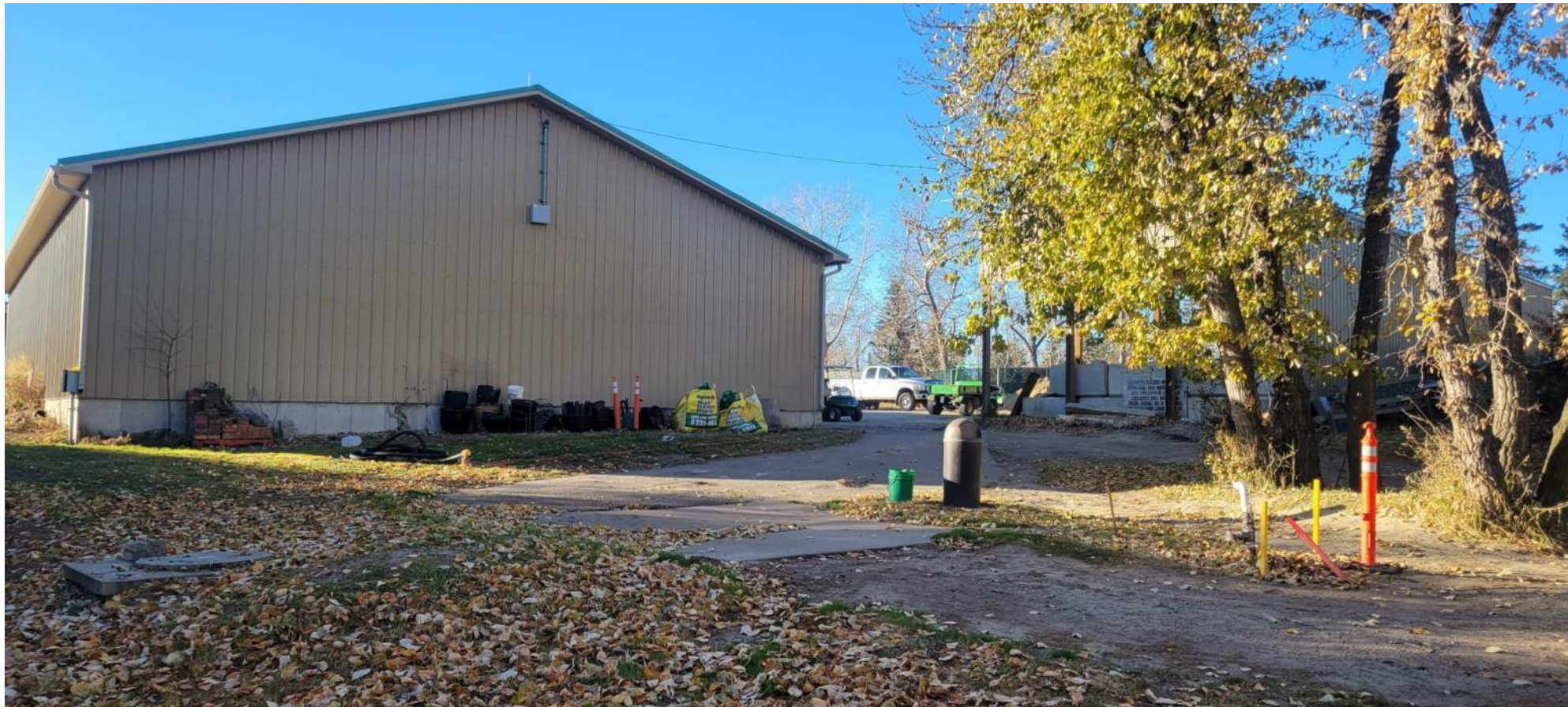
View from north looking south across building site area to existing maintenance area
