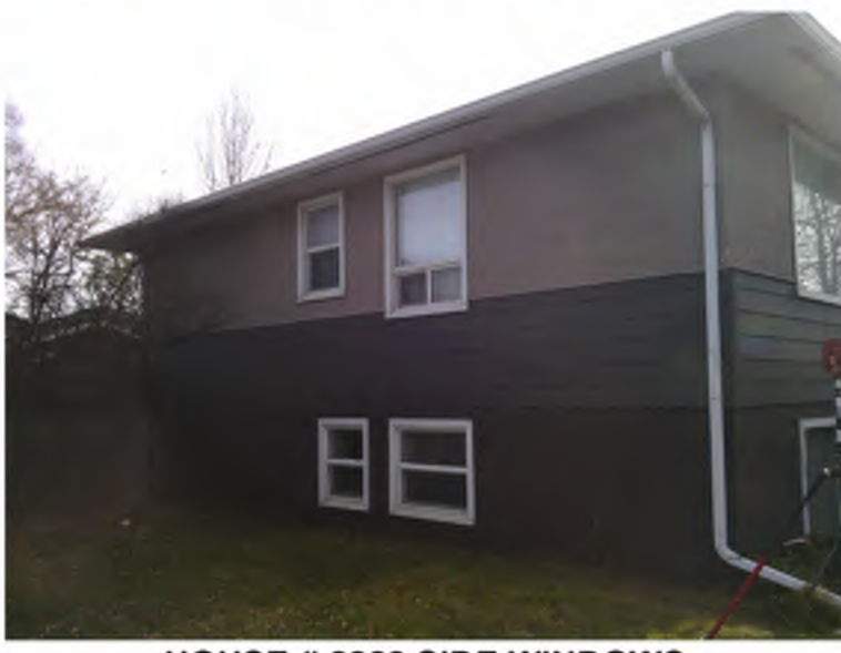
HOUSE # 2228 SIDE WINDOWS
