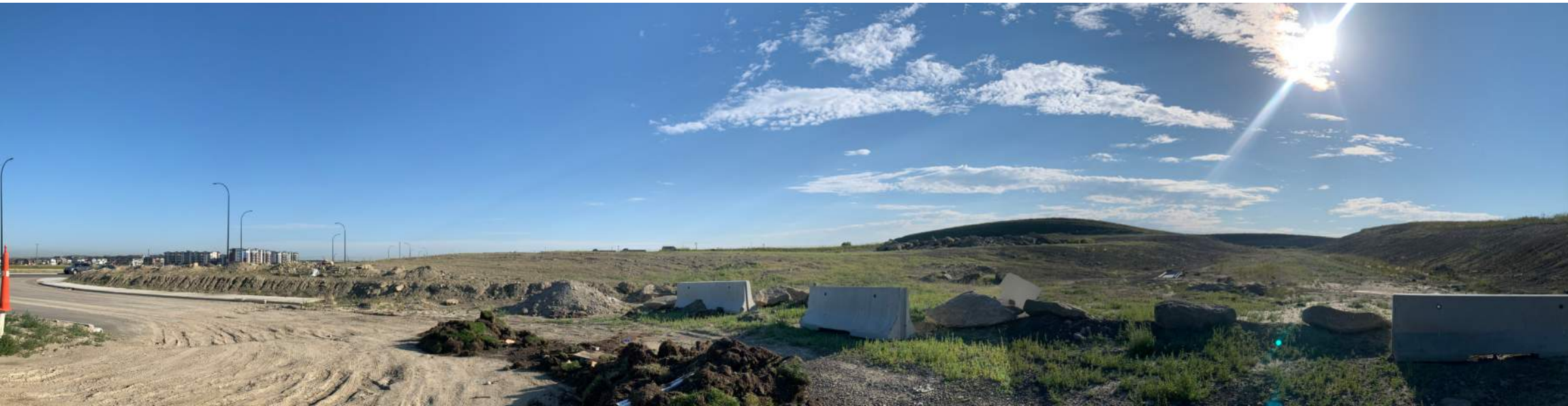
1. SITE IMAGE- SOUTH WEST CORNER LOOKING NORTH EAST
