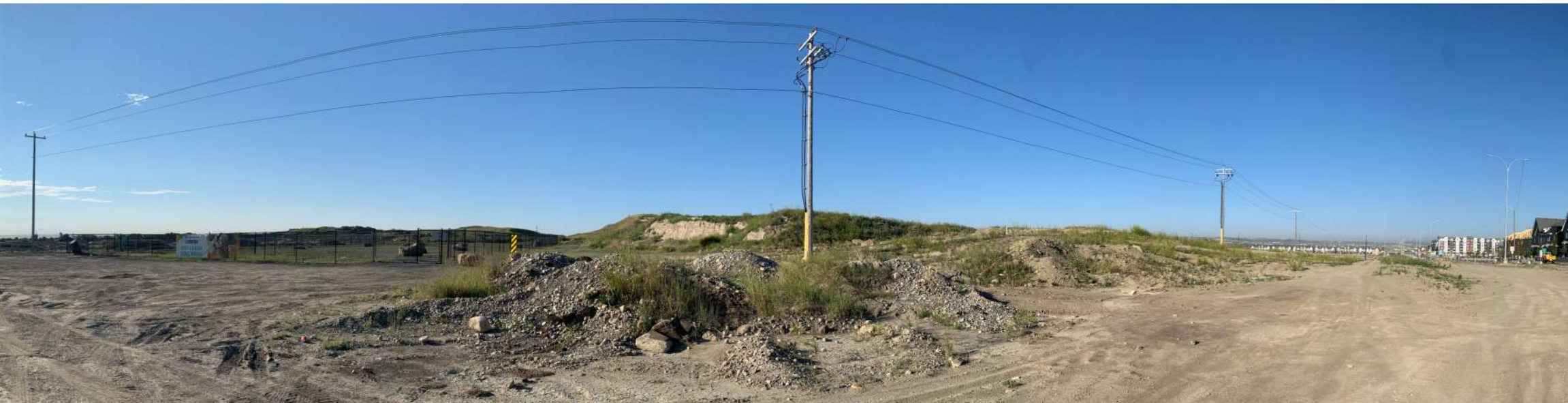
3. SITE IMAGE- NORTH EAST CORNER LOOKING SOUTH WEST
