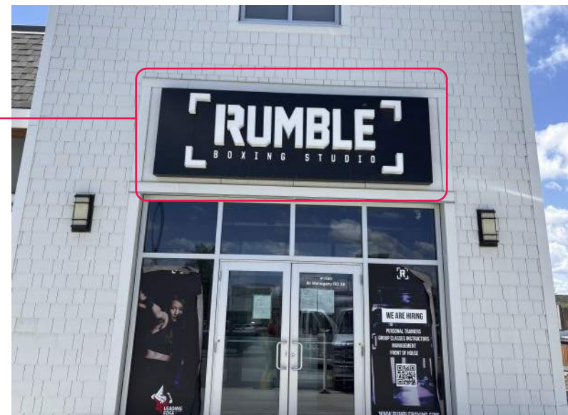
SHOWING EXISTING SIGN CABINET
