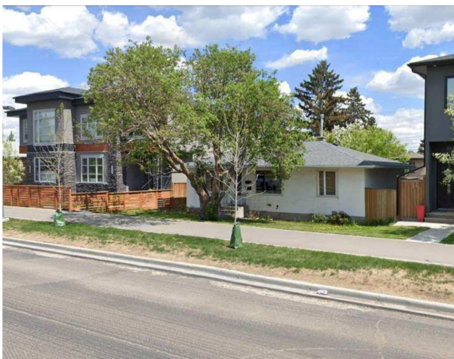
VIEW 3 - SW CORNER
