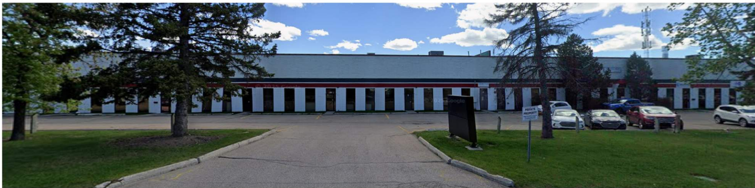
EXISTING NORTH (FRONT) OF BUILDING
