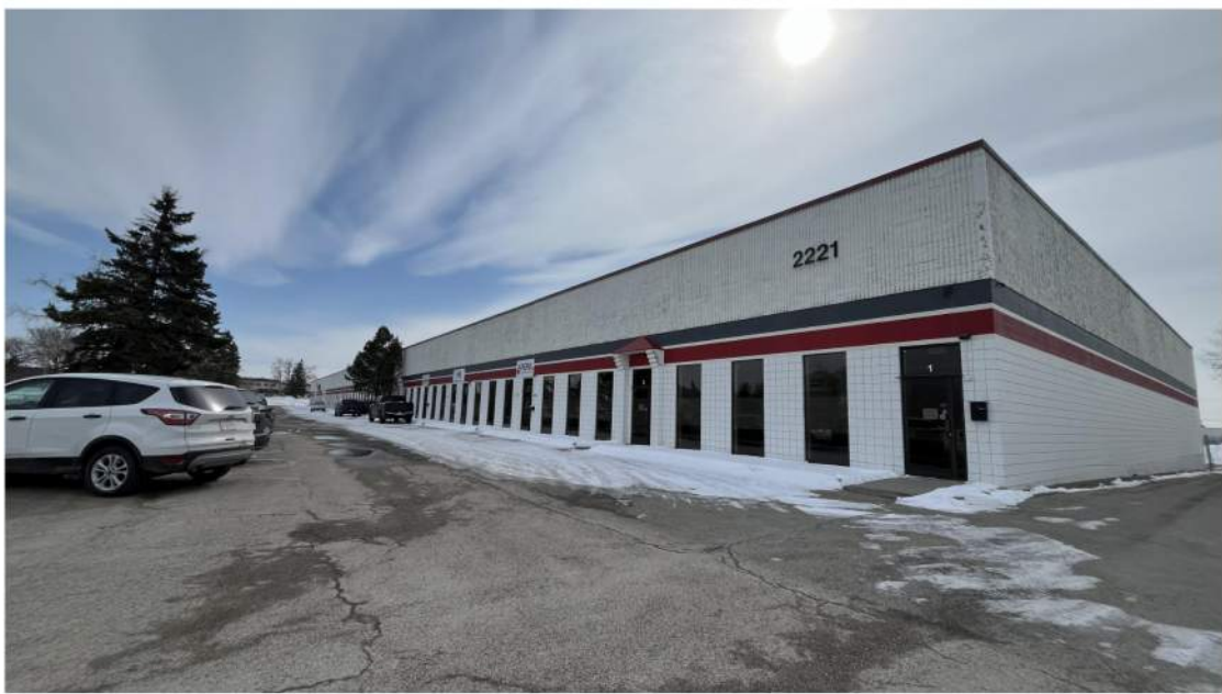
EXISTING NORTH (FRONT) & WEST (SIDE) OF BUILDING
