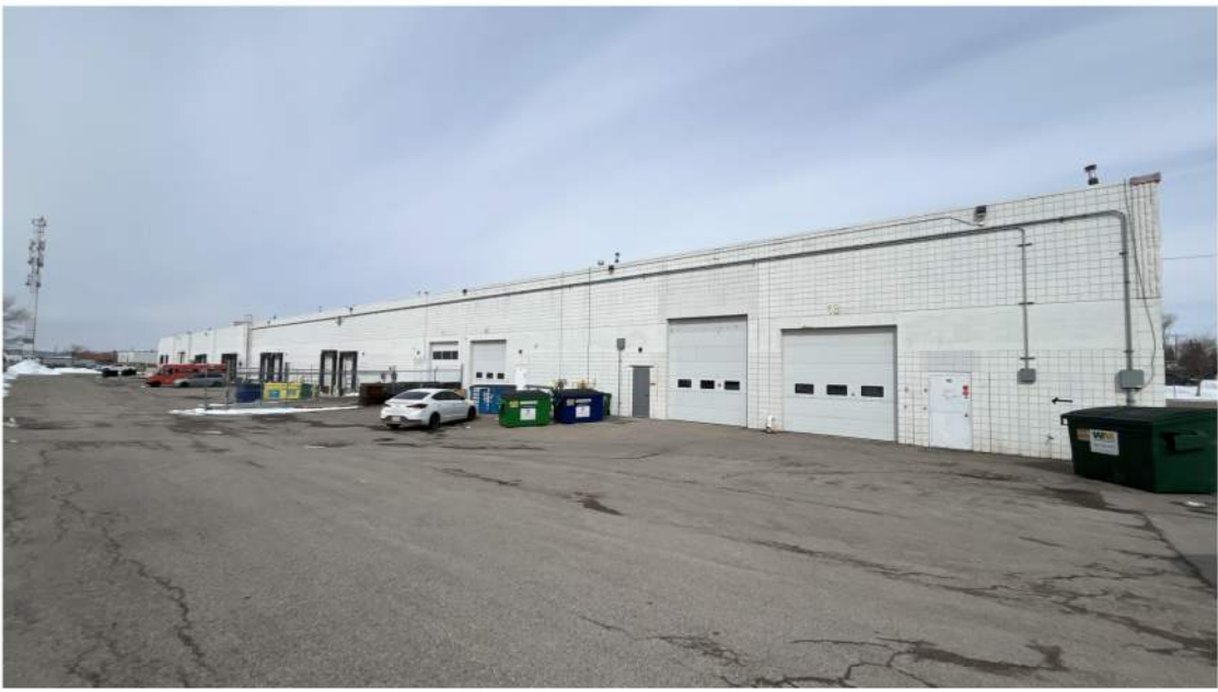
EXISTING SOUTH (REAR) OF BUILDING : NO CHANGES
