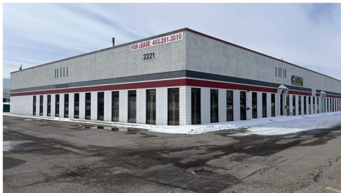
EXISTING EAST (SIDE) & NORTH (FRONT) OF BUILDING
