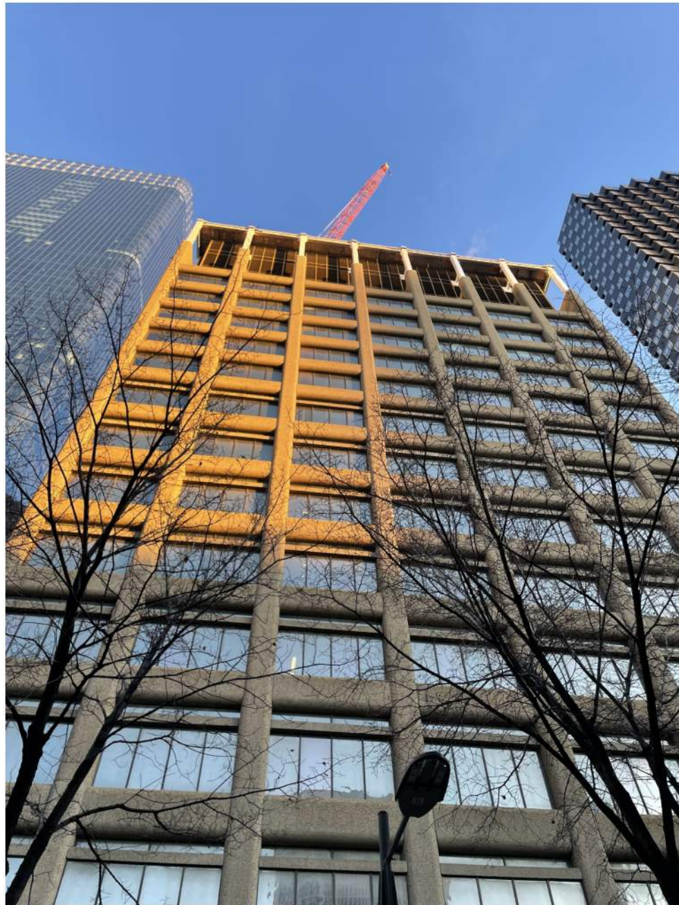
02 VIEW 2 VIEW WITHIN 30M SOUTH OF PROPERTY LINE NTS
