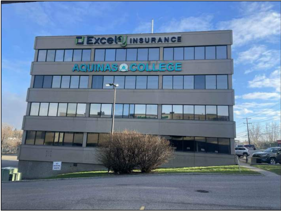
EXISTING SITE - VIEW FROM BUILDING B PARKING
