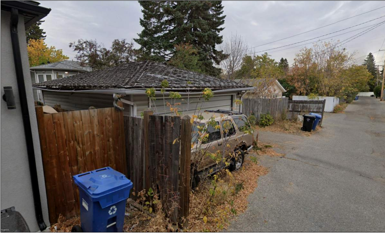
5. SOUTH WEST VIEW
