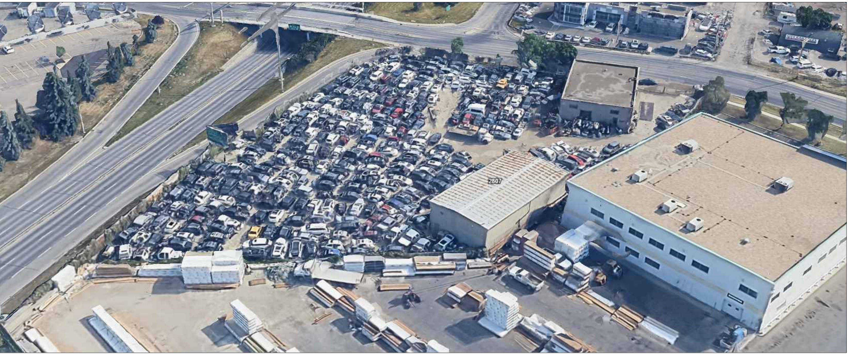
5 DP001 AERIAL PHOTO - SW CORNER SCALE: NTS
