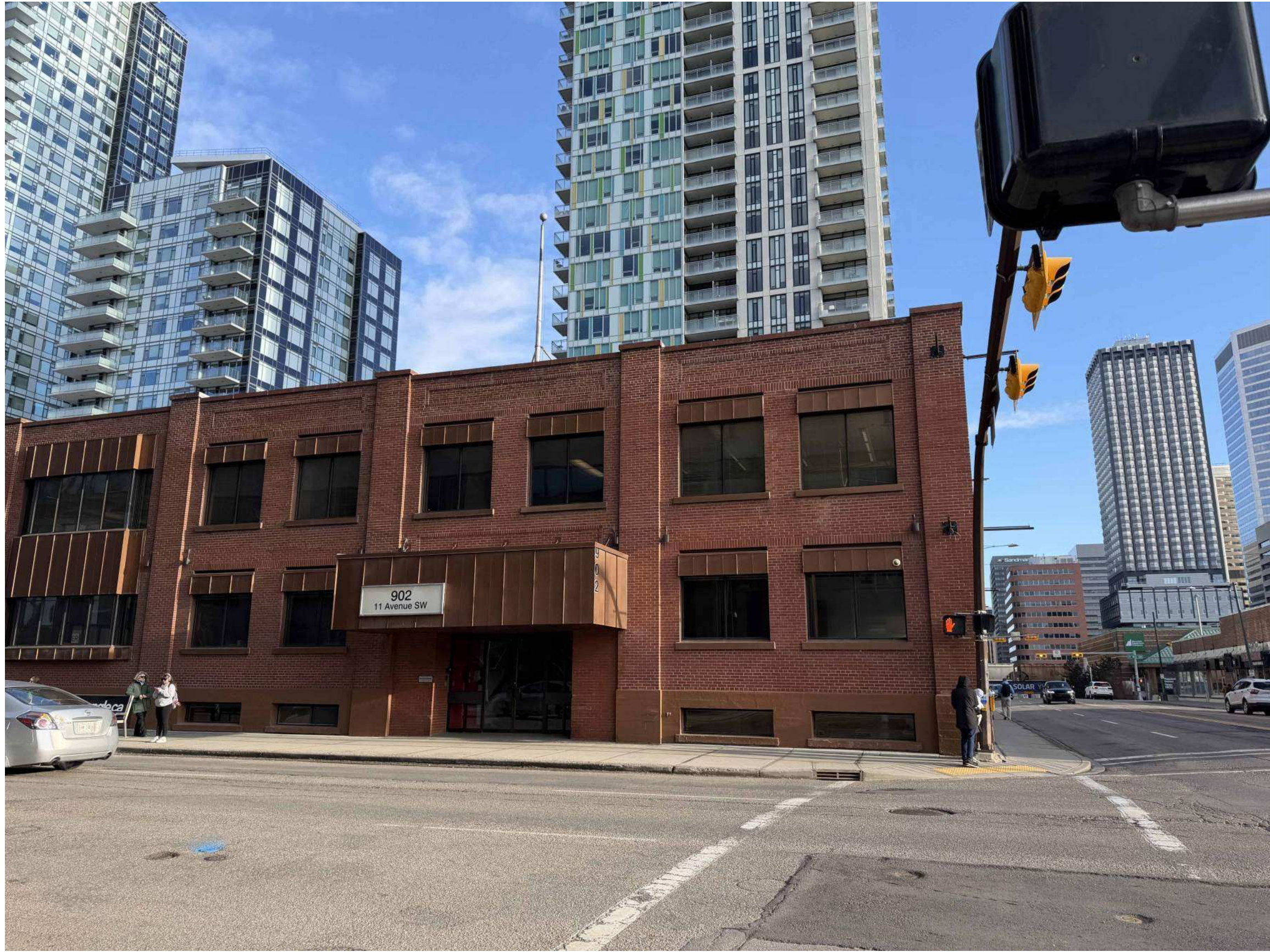
2 SOUTH VIEW DP.03
