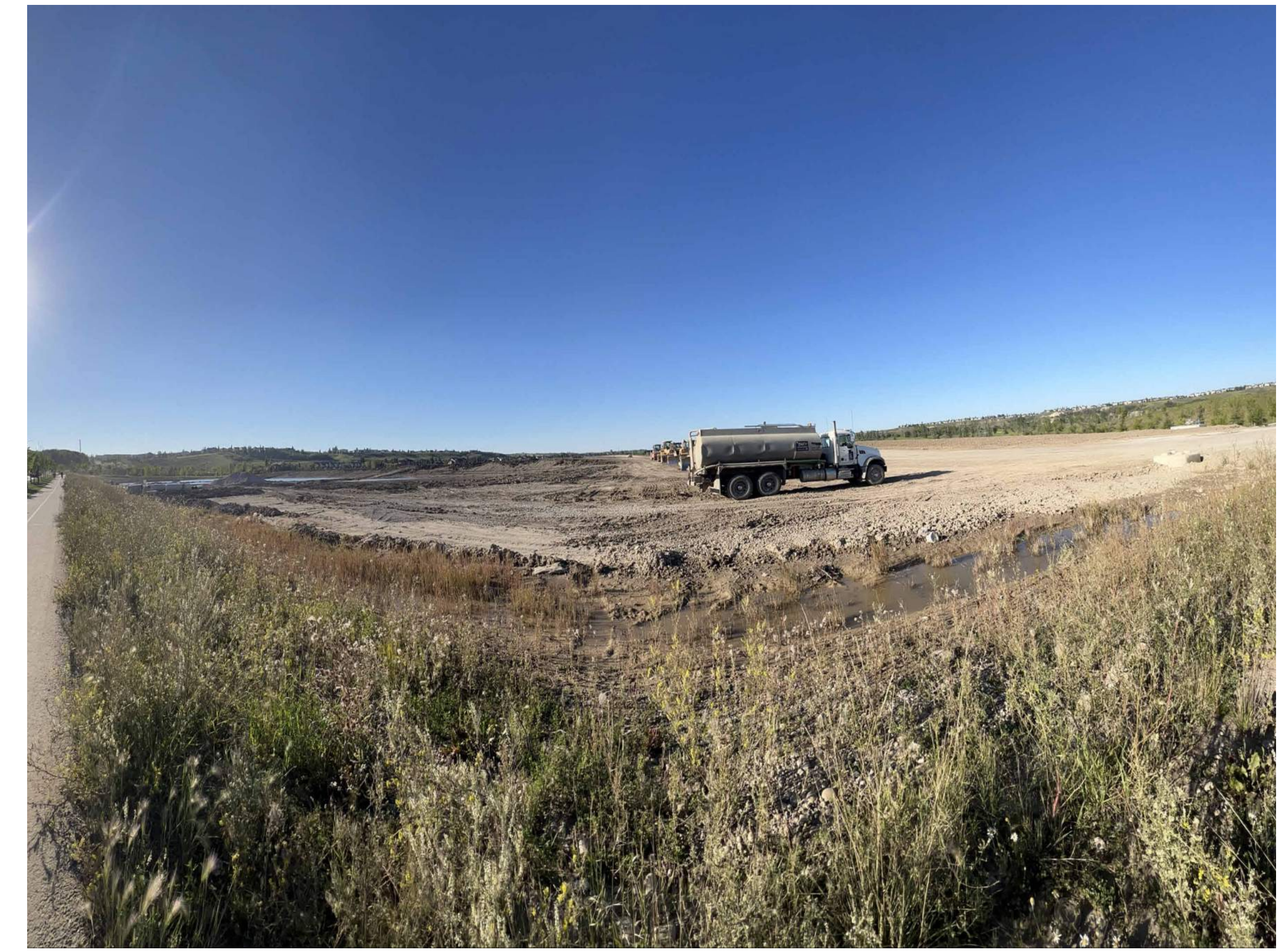
SITE PHOTO 3 - S VIEW SCALE: 1 : 250
