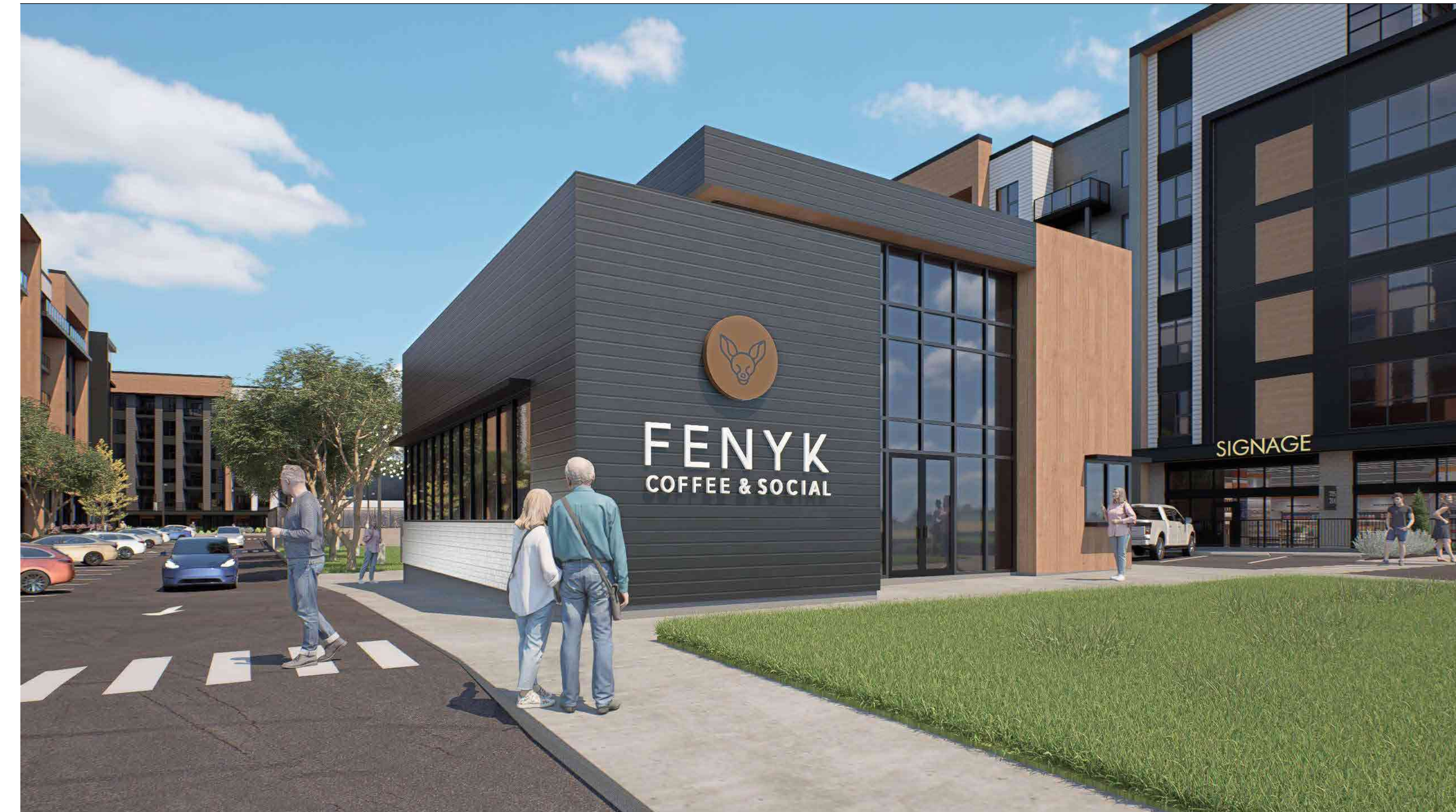
FROM BUILDING 3 CORNER
