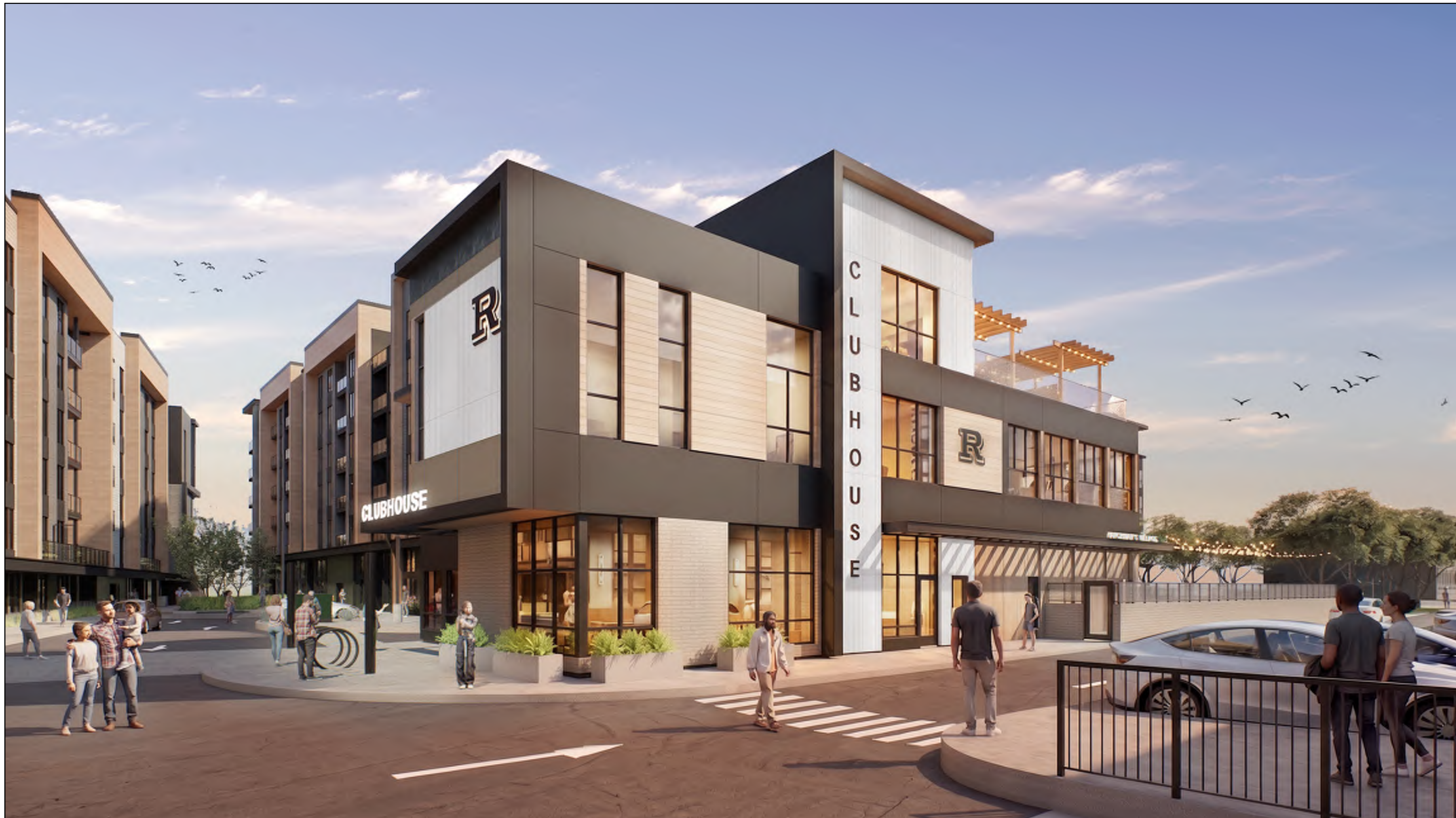
FROM BUILDING 3 CORNER
