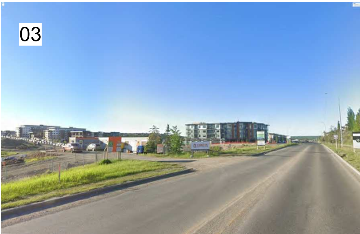
03 NORTH-WEST OF SITE - LOOKING SE ALONG 85th ST SW
