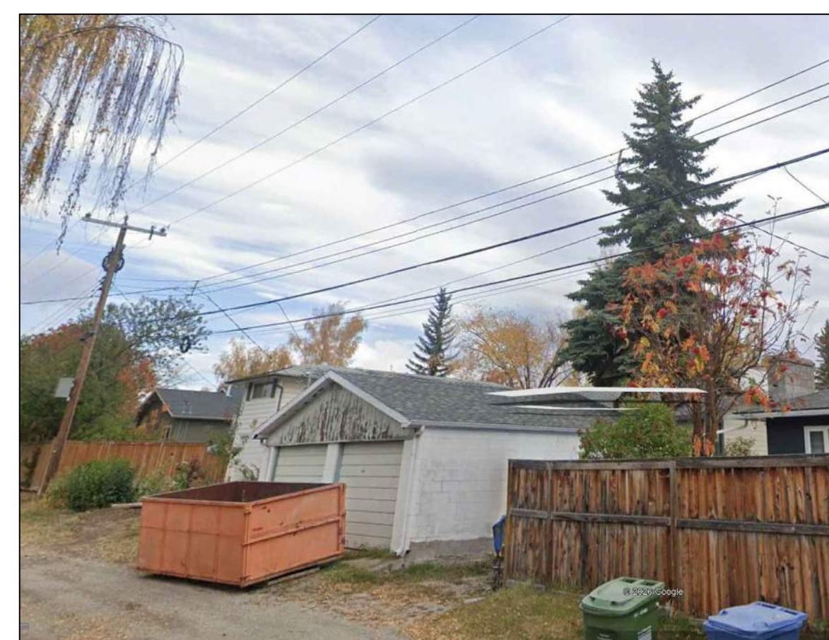
Rear yard garage taken from lane (south elevation)
