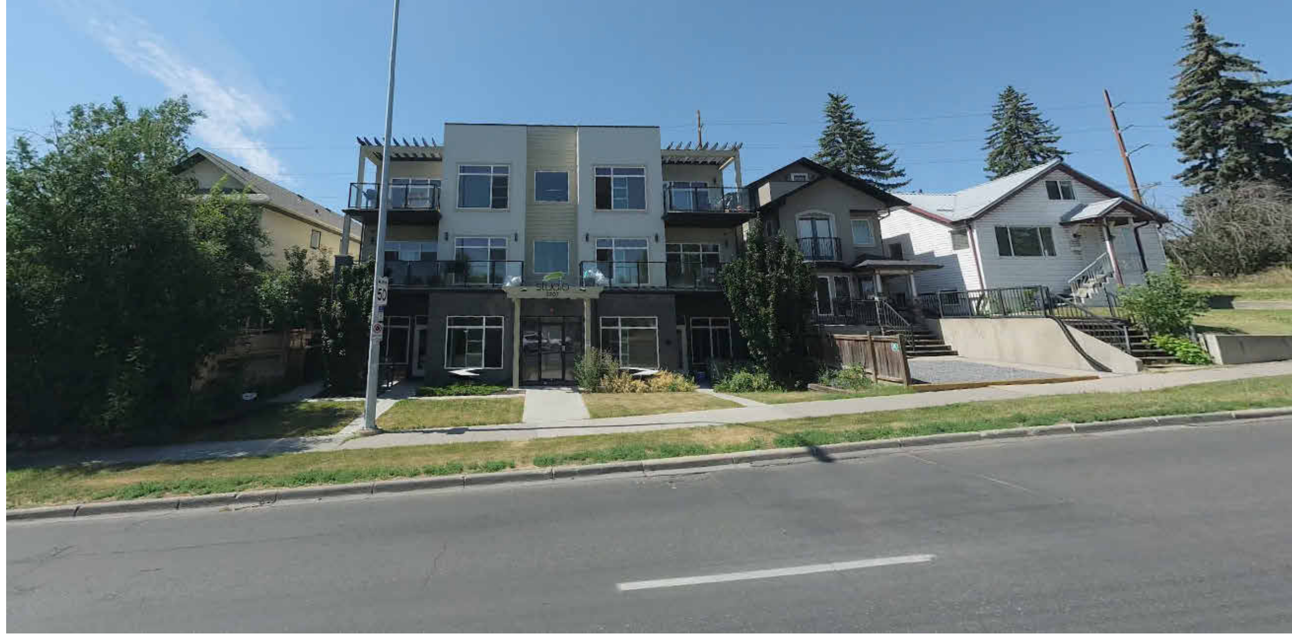
SP 4 - SITE PHOTO - CENTRE STREET N LOOKING EAST
