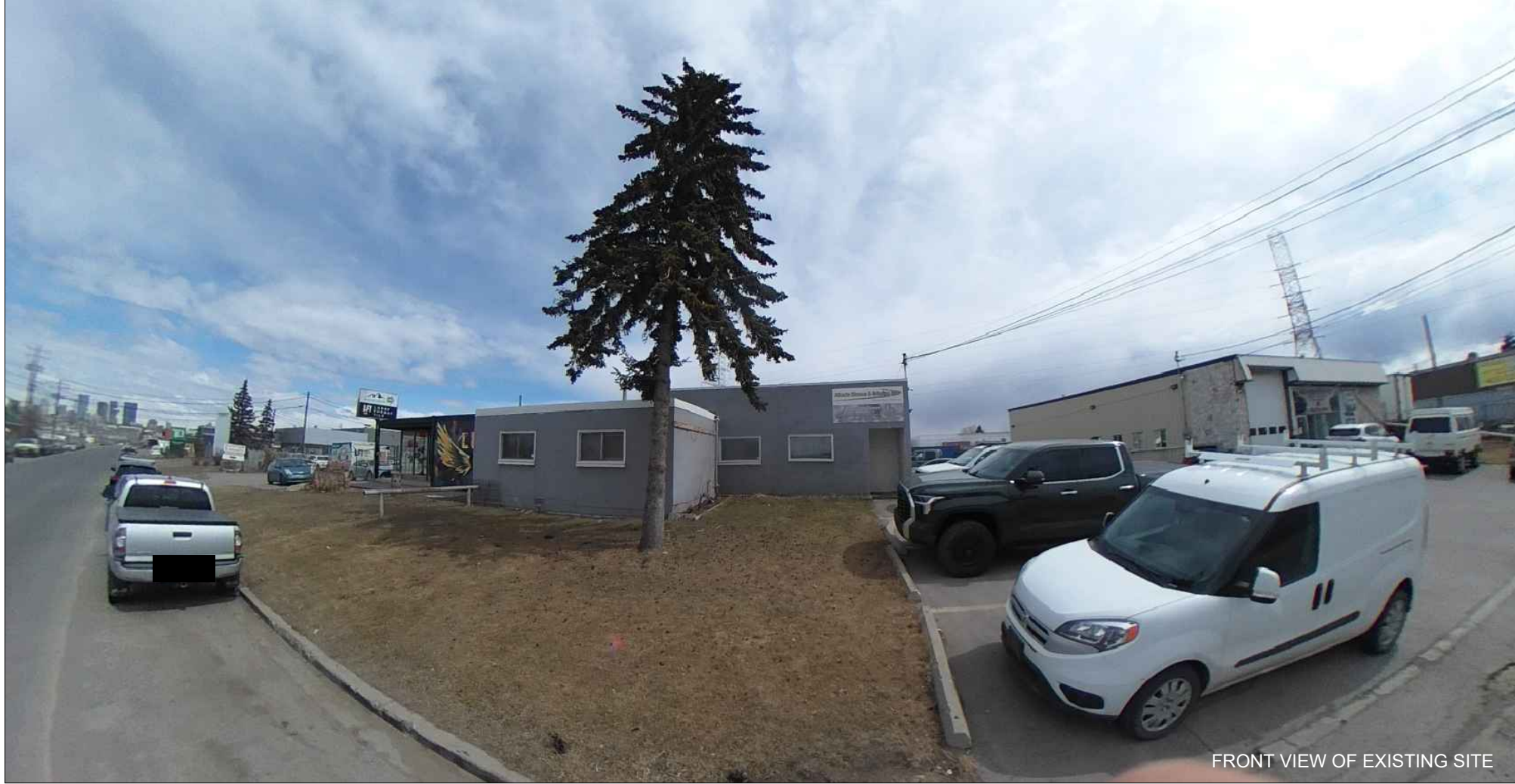
FRONT VIEW OF EXISTING SITE
