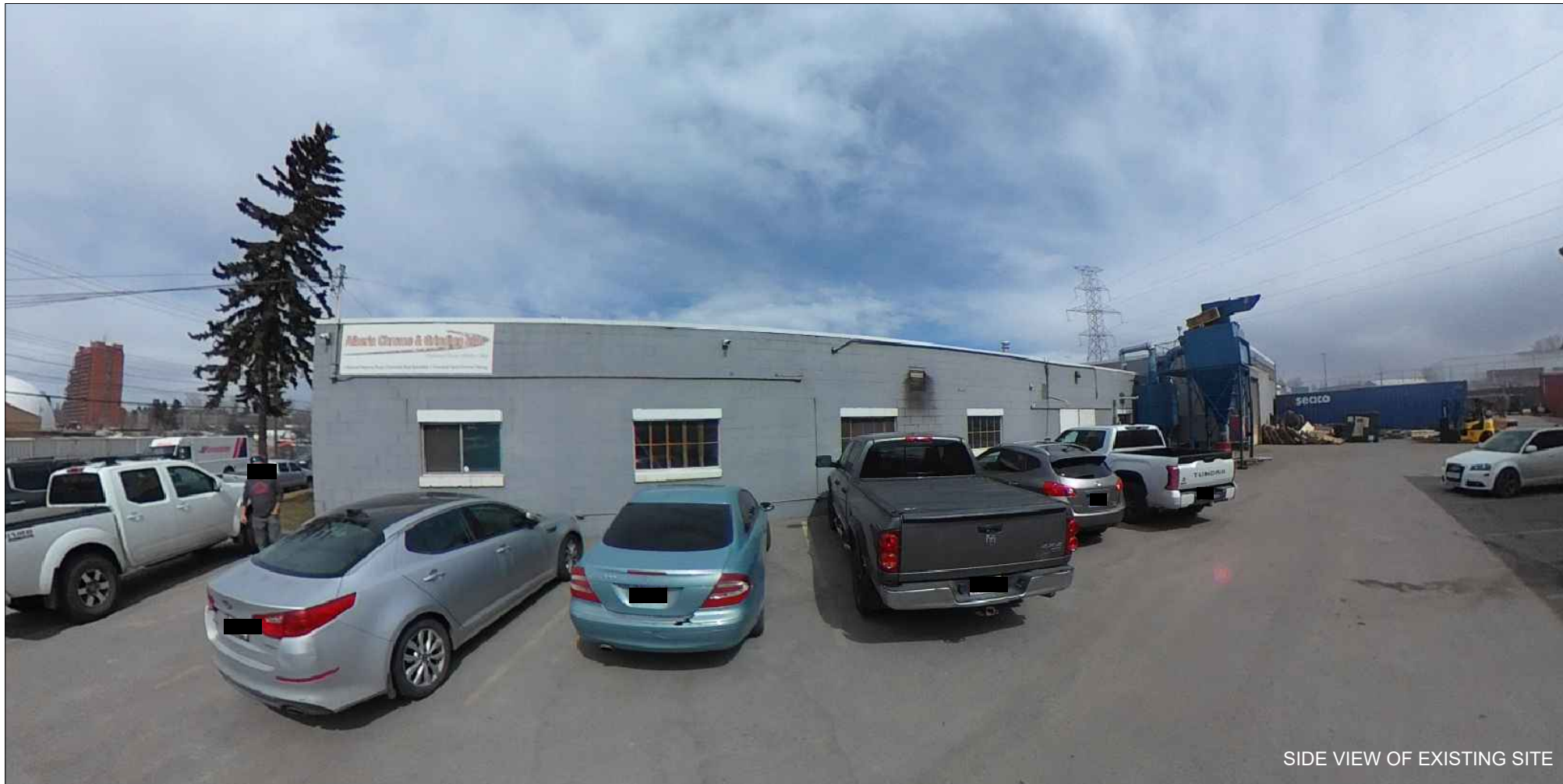
SIDE VIEW OF EXISTING SITE
