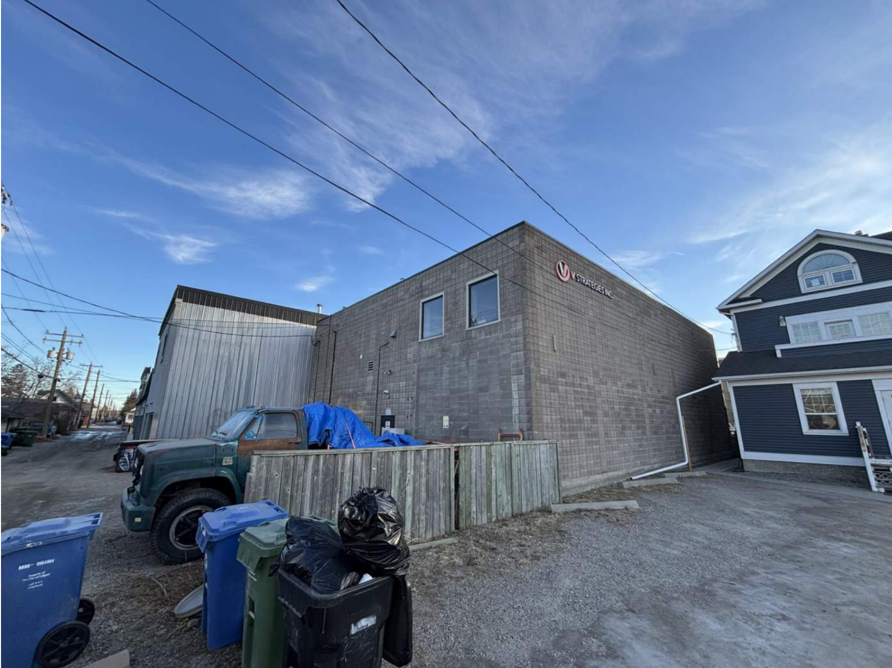
NORTHWEST CORNER OF PROPERTY
