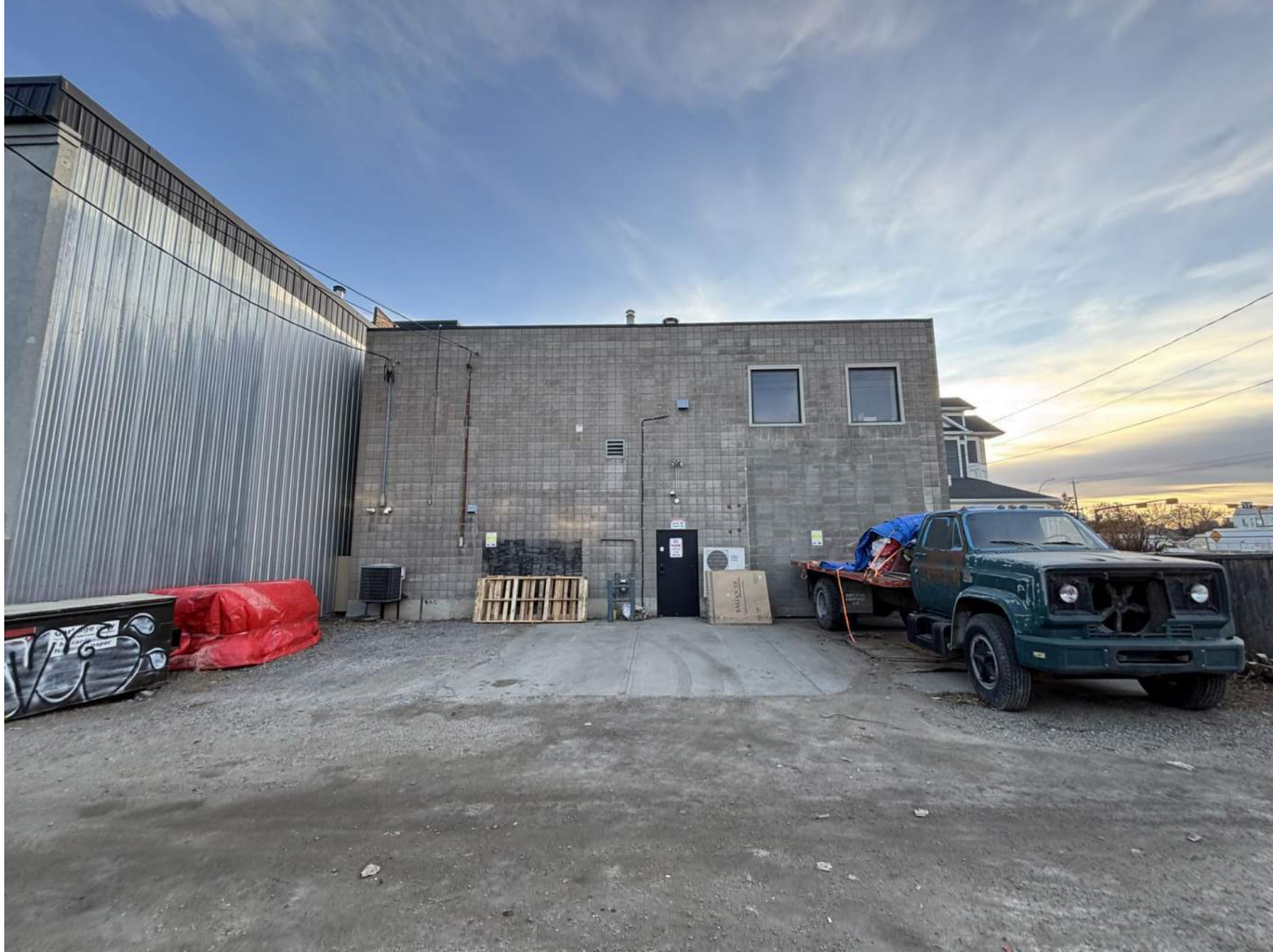
NORTH FACADE FROM REAR LANE
