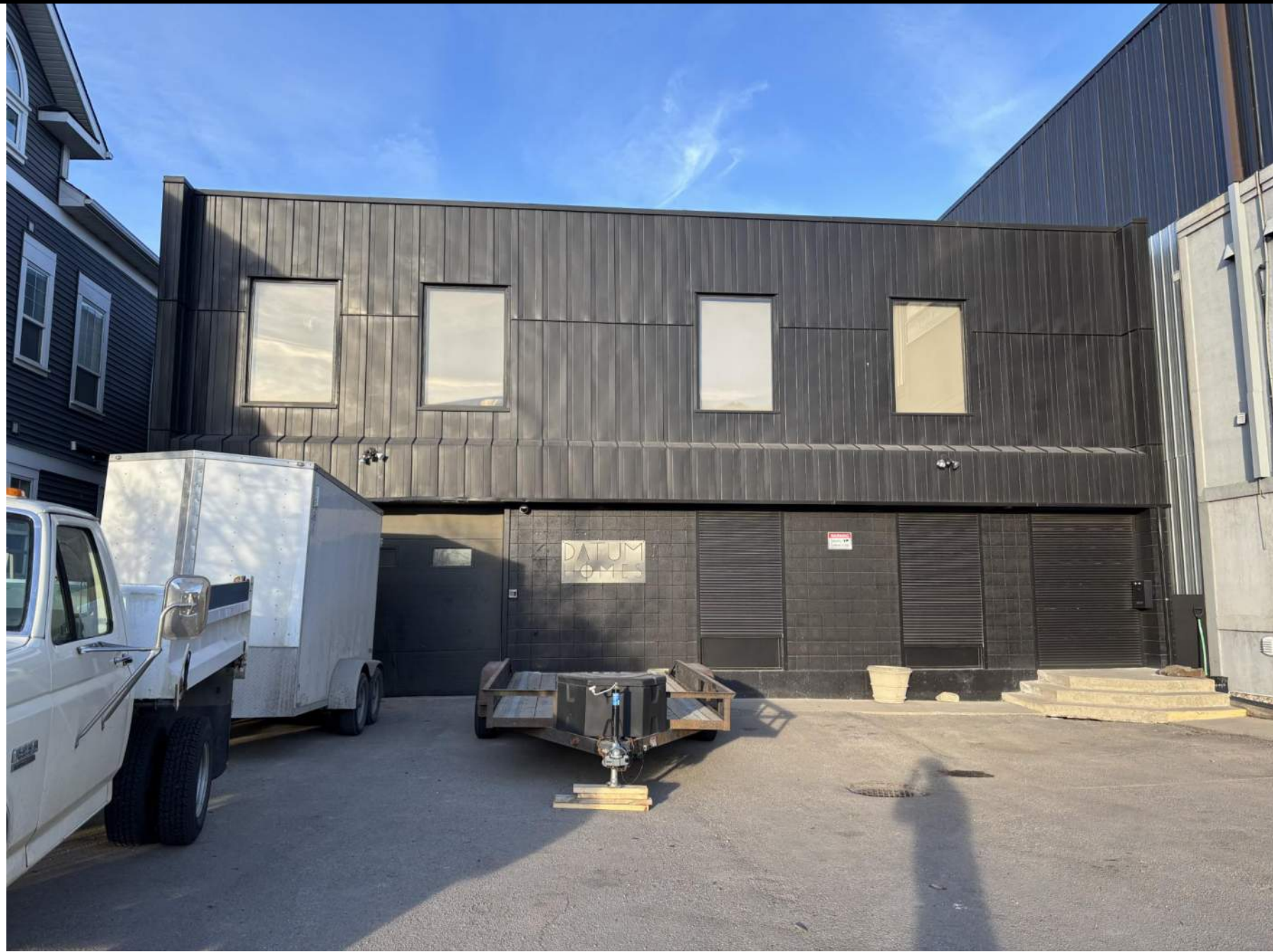
SOUTHWEST CORNER OF PROPERTY
