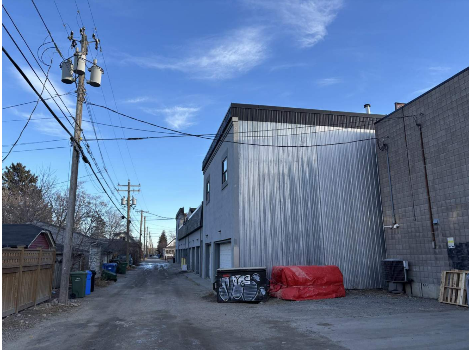
OVERHEAD POWER LINE/POLE
