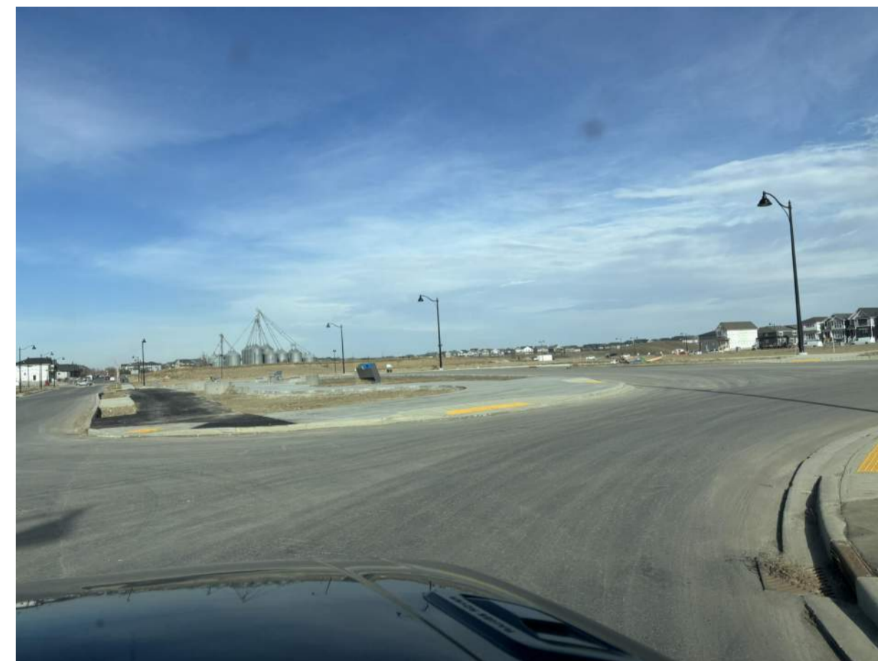
EXISTING SITE IMAGE 01 - LOOKING NORTH
